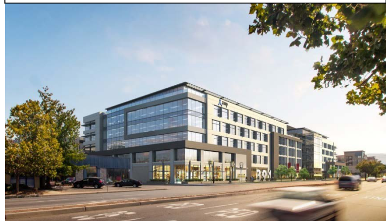
View of Building 2 from San Antonio Road
