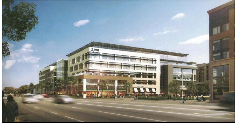
View of Building 1 from San Antonio Road
