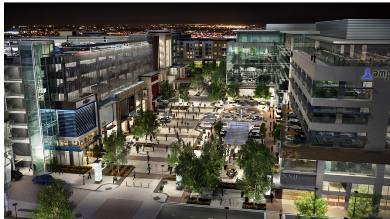
View of Building 5 Parking Structure, Central Plaza, and Office Buildings from the North
