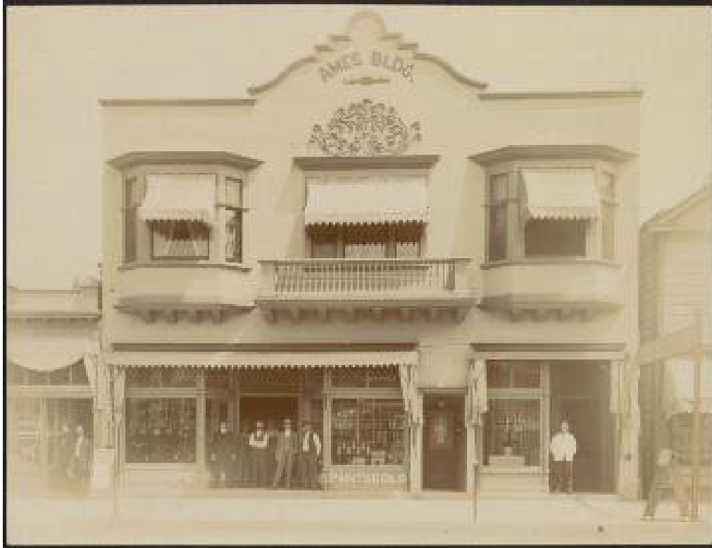
Figure 9. Ames Building 1907, after 1906 earthquake; note one-story addition to north side of building. Mountain View Hardware Company and Club Restaurant (Leo Miller, proprietor in doorway) shown. A.L. Boynton Electrical Supplies to left of hardware store (Source: City of Mountain View Public Library, Call # PHA B4 8).
