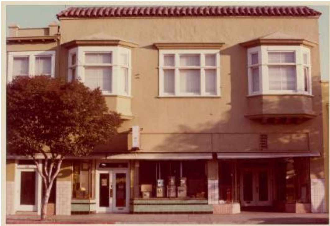
Figure 10. Ames Building 1976, showing alterations to storefront, roofline, balcony, and two-story addition to north side of building (Source: City of Mountain View Public Library, Call # PHA B4 9).
