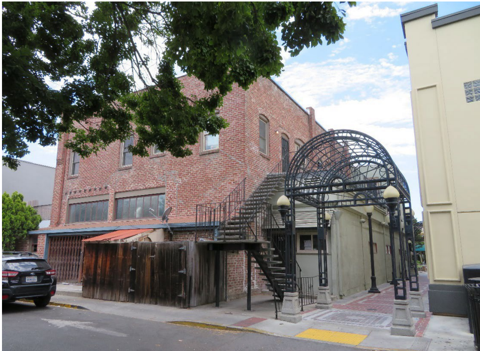
Figure 19. Existing conditions at rear façade, view southwest, June 2022 (ARG).
