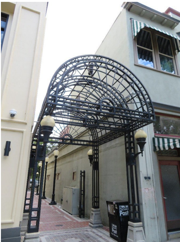
Figure 16. Existing conditions at north façade/alley, June 2022 (ARG).
