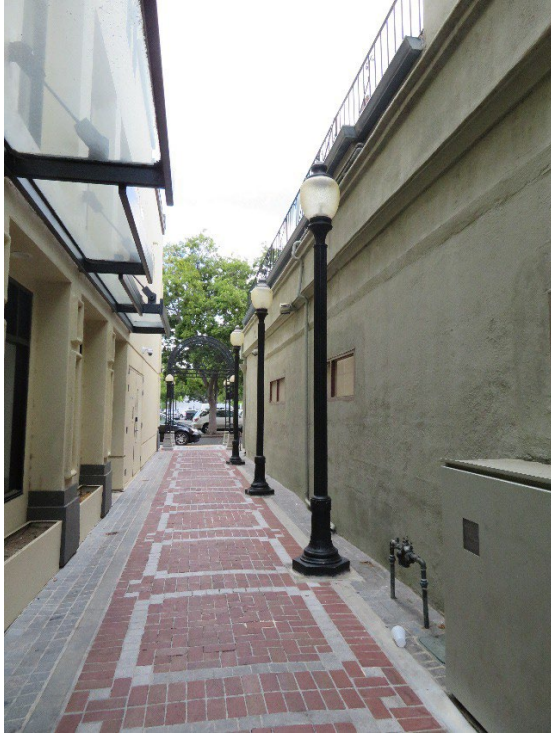
Figure 17. Existing conditions at north façade/alley, looking southeast, June 2022 (ARG).
