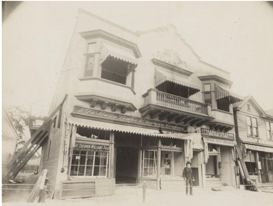
Figure 7. Front of Ames Building following 1906 Earthquake (Source: City of Mountain View Public Library, Call # PHA B4 6).
