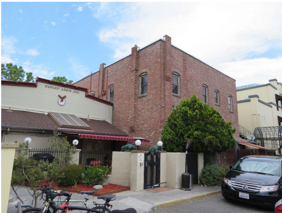
Figure 20. Existing conditions at rear façade, view northwest, June 2022 (ARG).
