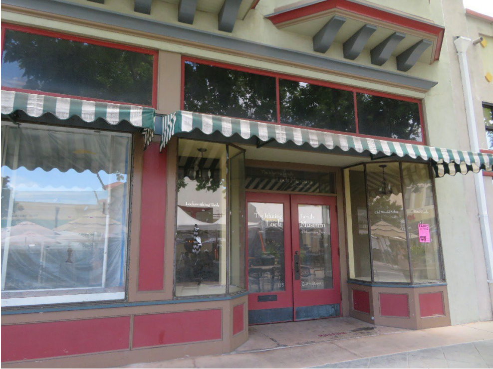
Figure 13. Existing conditions at southernmost storefront, June 2022 (ARG).
