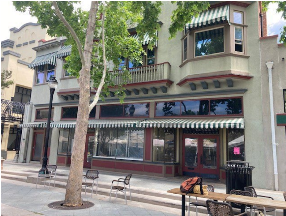
Figure 11. Existing conditions, front façade, June 2022 (ARG). Note: a communication from the Mountain View Historical Society indicates that the top half of the building's Castro Street façade was restored c.2003 to its original appearance (the parapet, false balcony, and decorative plasterwork were recreated).
