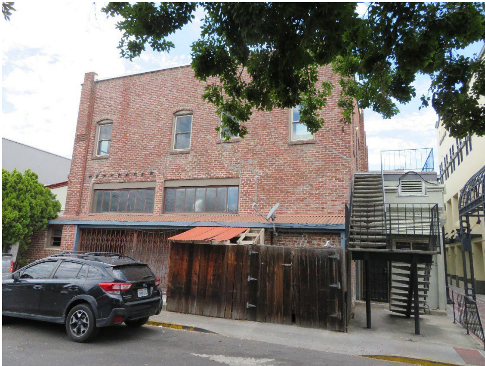
Figure 18. Existing conditions at rear façade, June 2022 (ARG).
