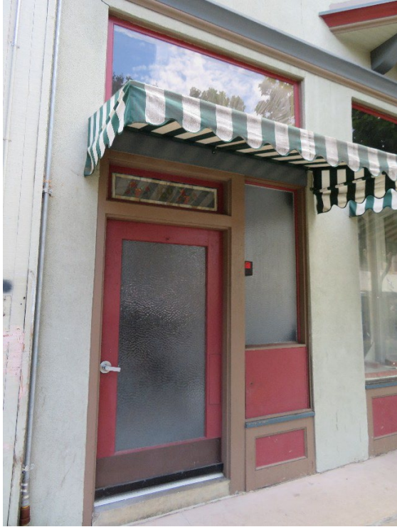
Figure 15. Existing conditions at storefront, northernmost entrance, June 2022 (ARG).
