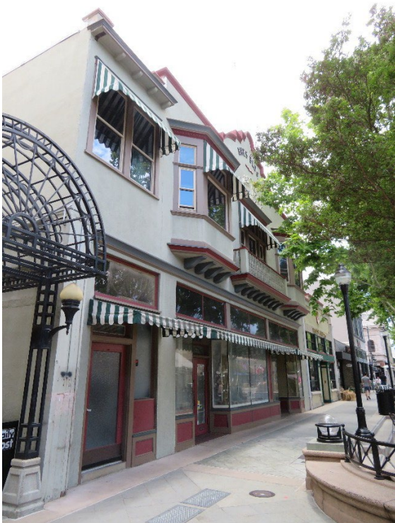
Figure 12. Existing conditions, front façade, June 2022 (ARG).
