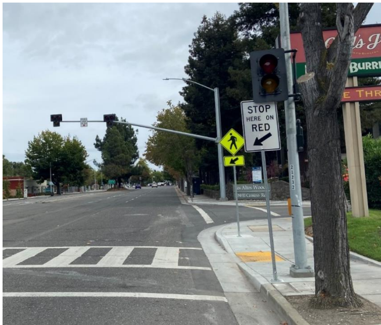
Figure 1: Pedestrian Hybrid Beacon at Distel Circle and El Camino Real, Mountain View
