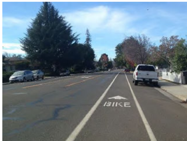
Figure 2-2 A standard bike lane on Cuesta Avenue includes painted edges lines, delineating the bike lane from the parking lane.
