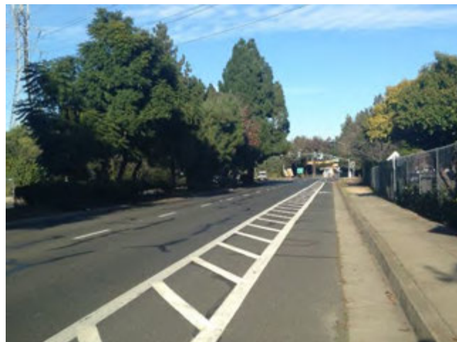
Figure 2-5 A buffered bike lane on Moffett Boulevard separates bikes from adjacent traffic.
