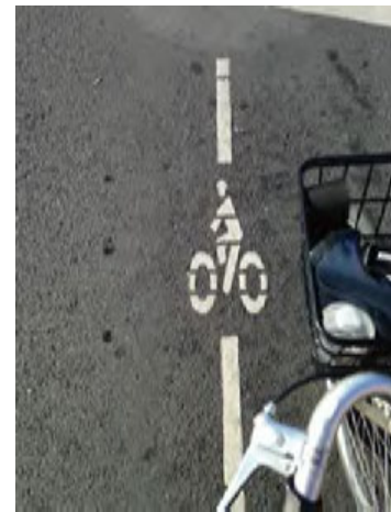
Figure 2-10 Bicycle detection pavement marking
