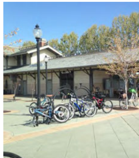
Figure 2-15 Class II bike parking at the Mountain View Transit Center.
