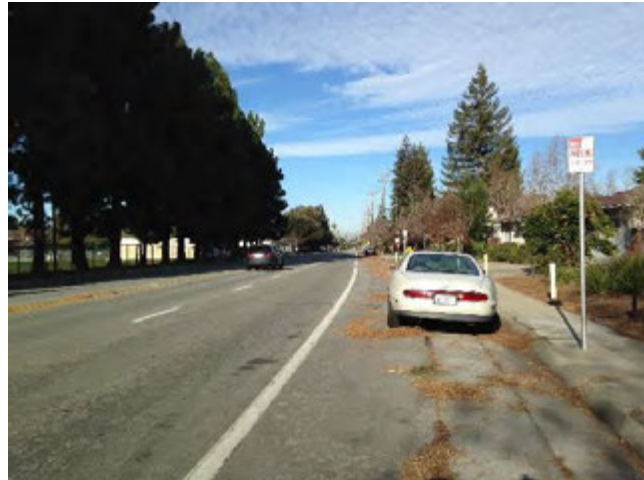
Figure 2-3 On North Whisman Road, the bicycle lane and parking lane share the same road space.
