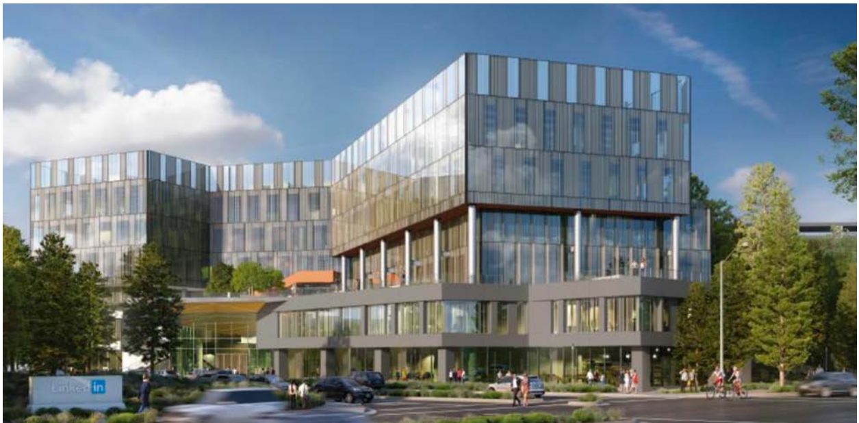
Glass curtain wall with visual interest
