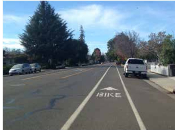
Figure 4-5 A standard bike lane on Cuesta Drive includes painted edges lines, delineating the bike lane from the parking lane
