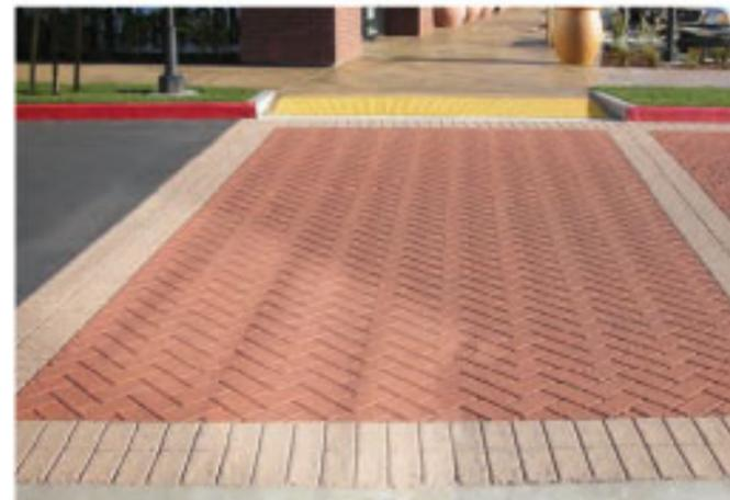
Vehicular Stamped Asphalt Paving
