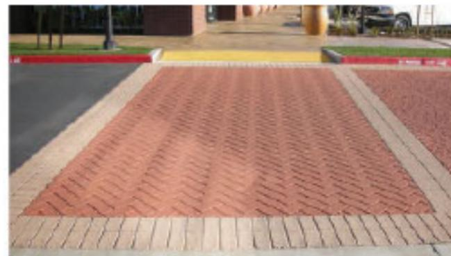
Vehicular Stamped Asphalt Paving
