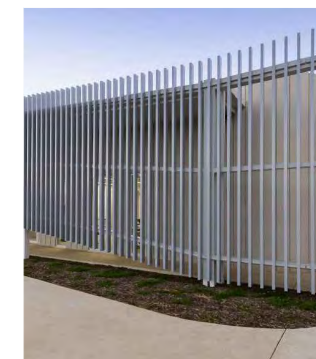
(MF) ALUMINUM METAL FINES @ PARKING GARAGE
