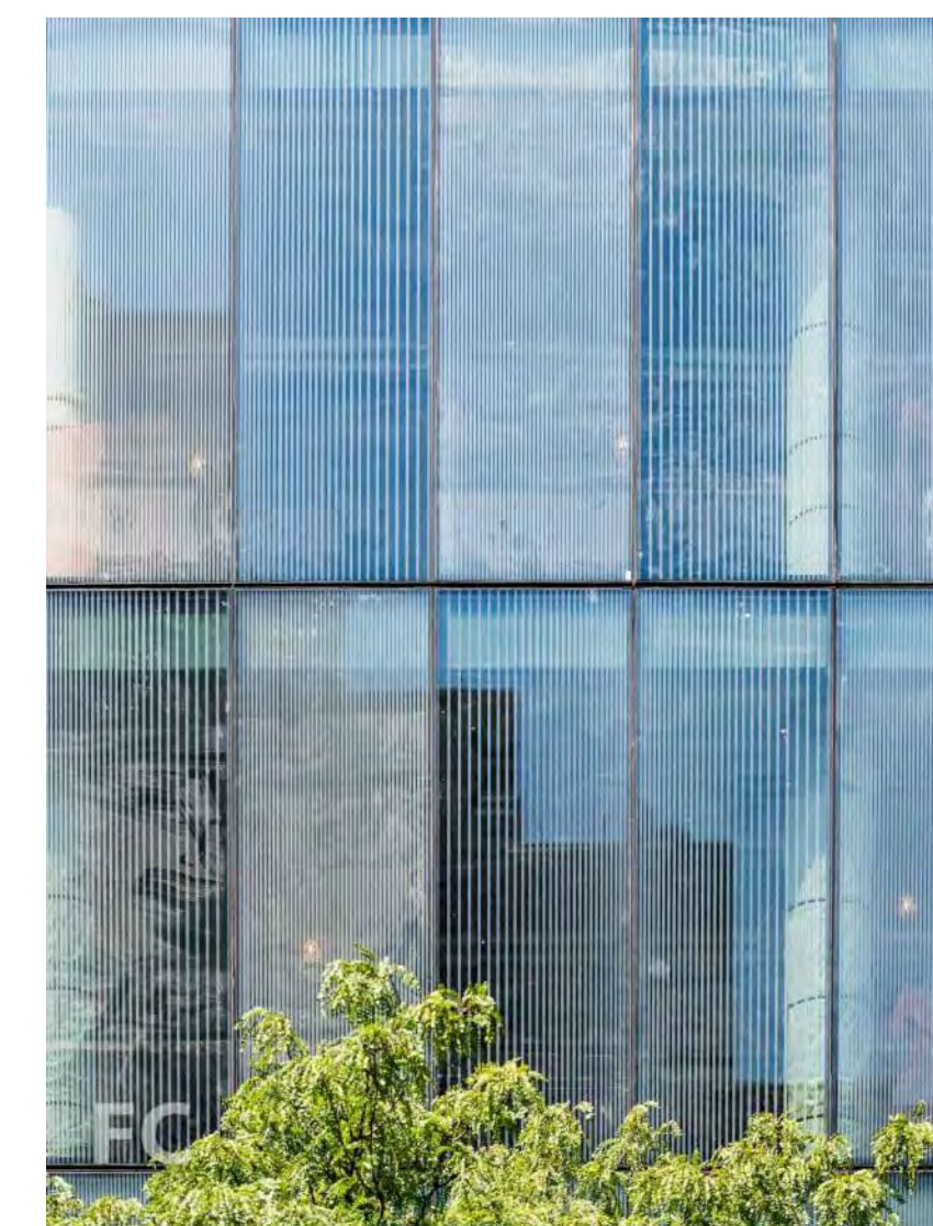
FRITTED GLASS AND VERTICAL FINES FACADE
