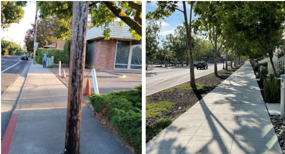
Figure 8 Examples of Different Sidewalk Conditions in Mountain View
