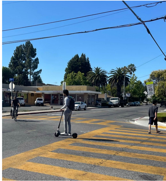
Marked crosswalks can help motorists anticipate the presence of people walking and biking at intersections.
