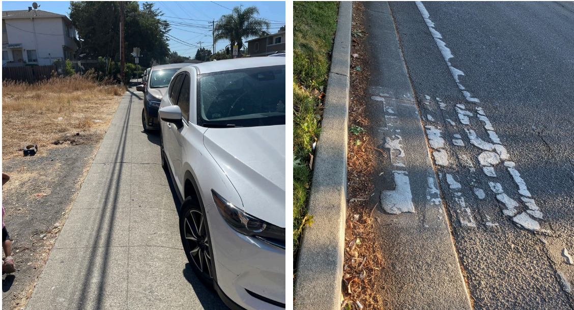
Figure 26 Example of a Rolled Curb and a Curb-Impacted Bike Lane in Mountain View
