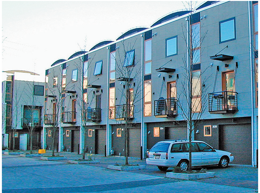
In order to provide enclosed two-car garages for each unit, stacked rowhouse projects typically utilize tandem parking for most units.
