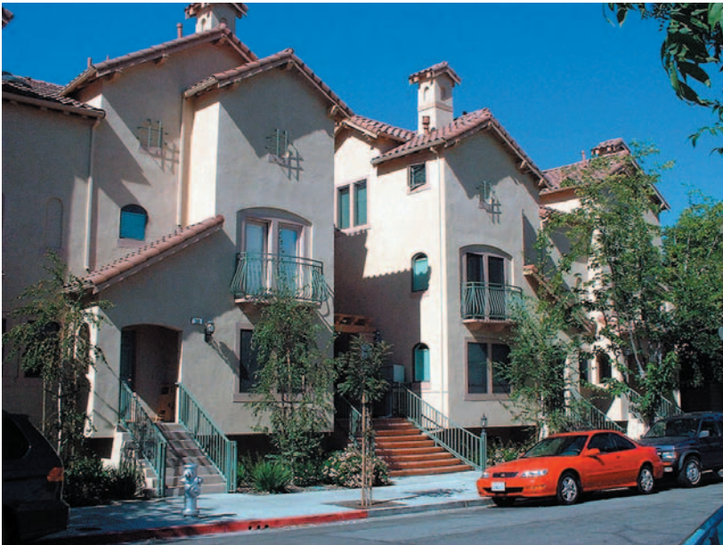
Stoops and balconies often project down from the units to the ground level to disguise the parking garage.
