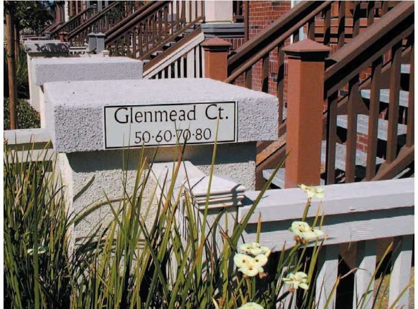
Building signage and address numbers should be clearly visible to visitors. Address numbers may also appear along driveways/alleys if buildings front on common open spaces or paseos.
