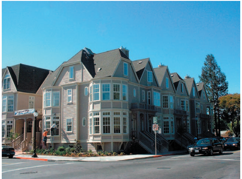
Podium Rowhouses in Downtown Mountain View
