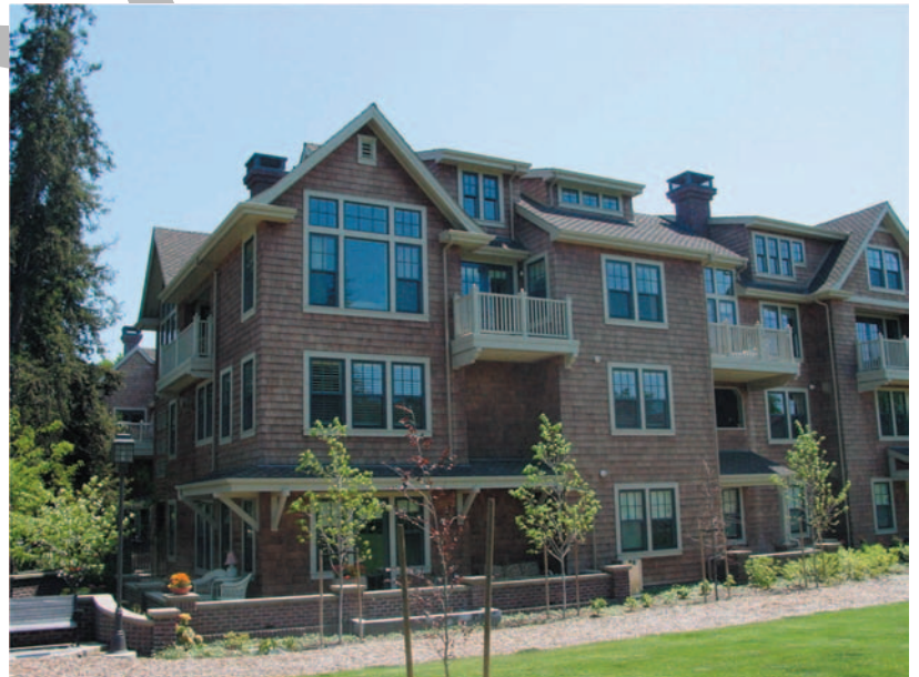
Long horizontal eaves and roof elements across the facade should be broken up with gables, building projections and articulation.
