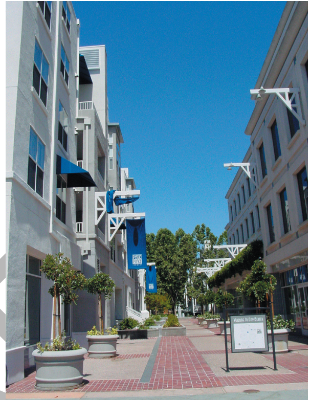
Multifamily development in the R4 zoning district shall have a maximum density of 60 du/ac. 80
