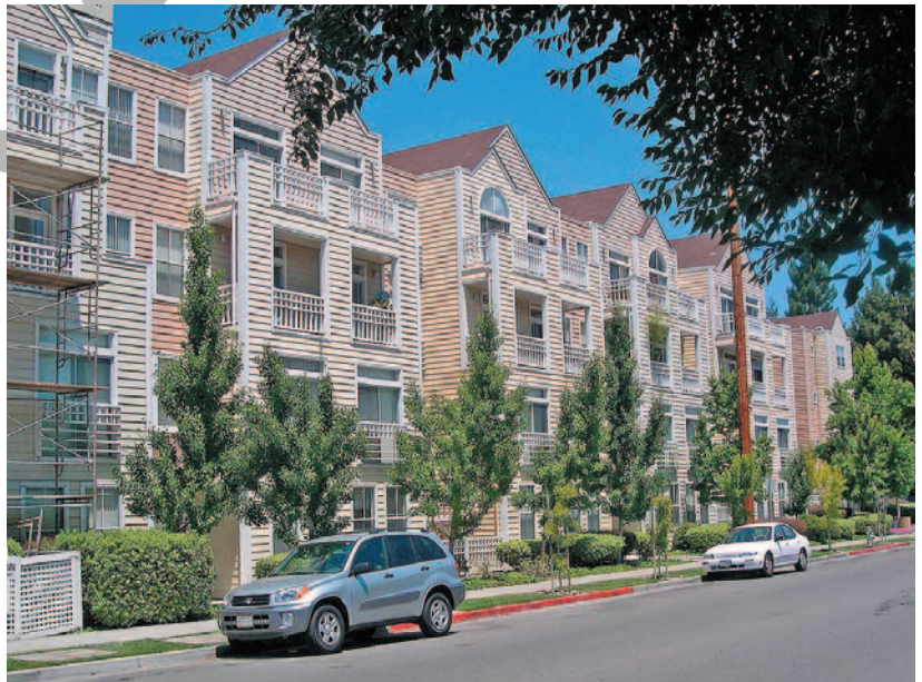
Stacked Flats in Downtown Mountain View
