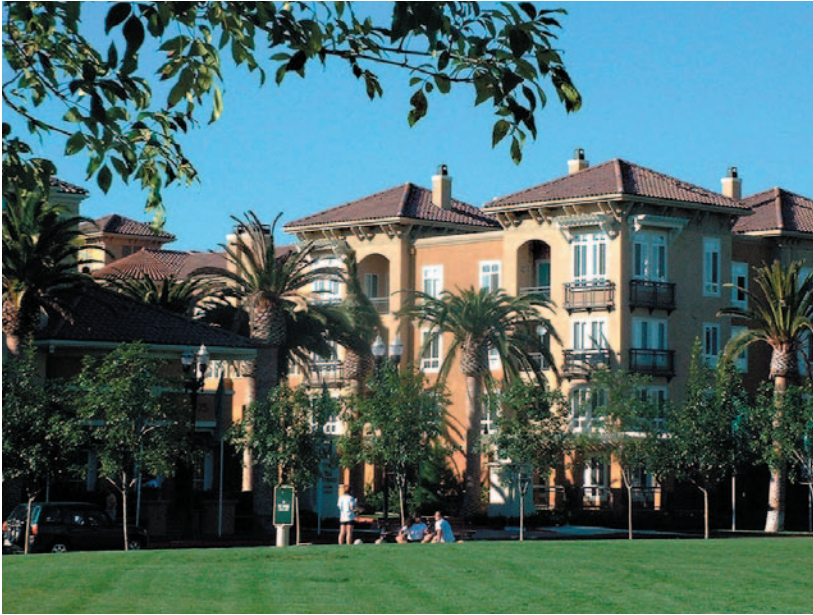
Multi-family developments should provide adequate, usable, safe and high quality common and private amenity areas.
