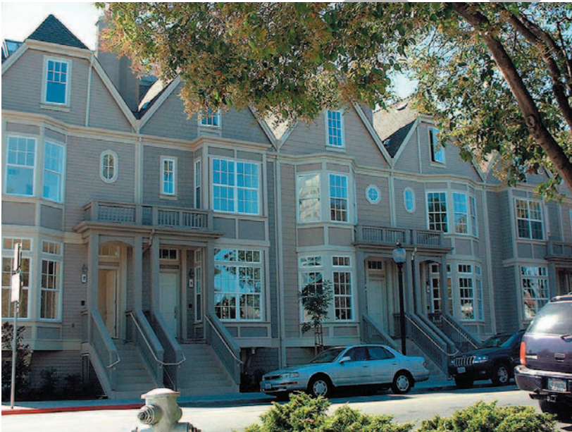
Recently built condominium projects on Bryant Street in Downtown Mountain View resemble rowhouses, but have stacked flats over the rowhouses and are built over a common submerged parking garage rather than with individual garages as part of each unit.
