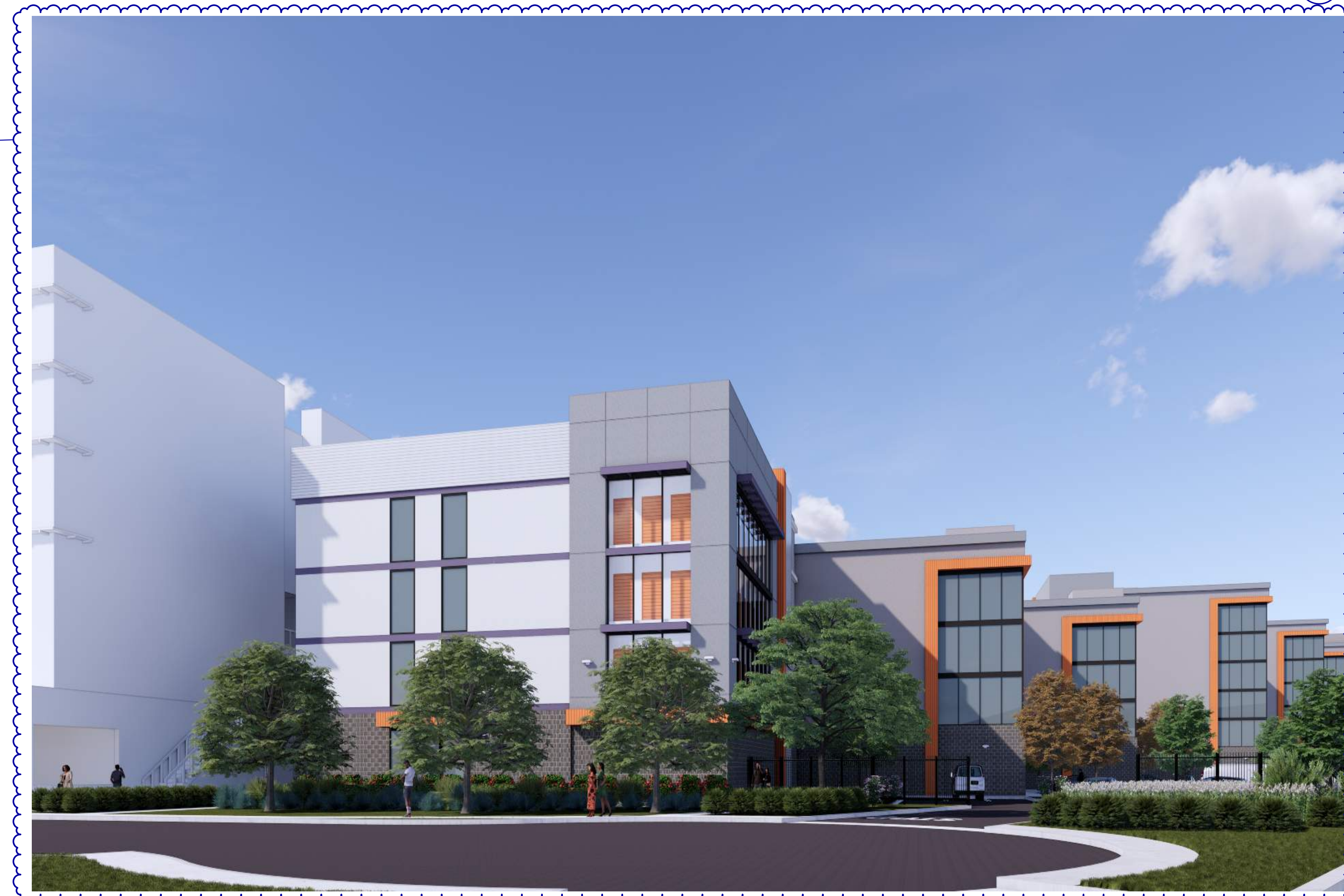
BUILDING 1 - SW CORNER VIEW
