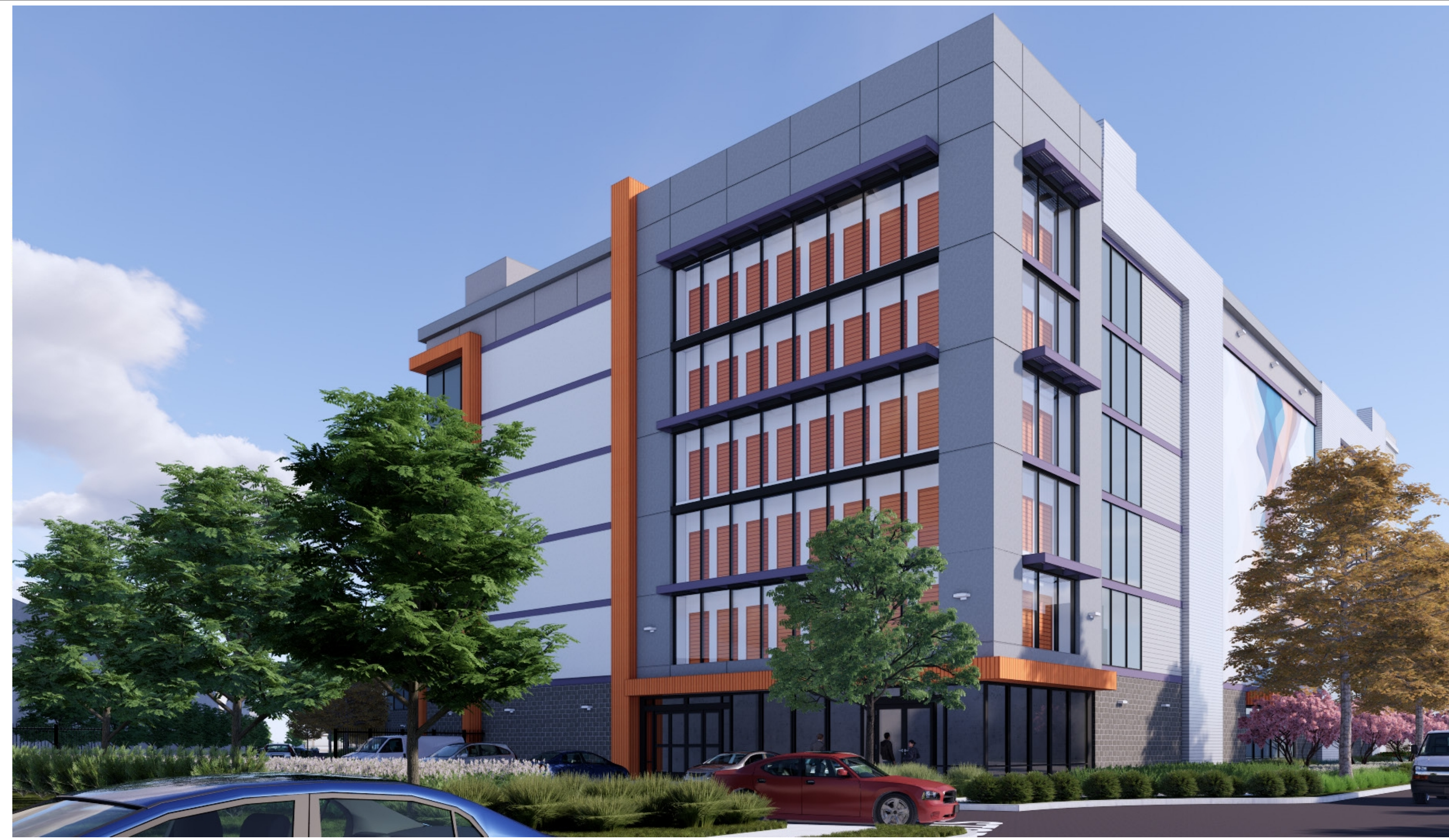
BUILDING 1 - NE CORNER VIEW
