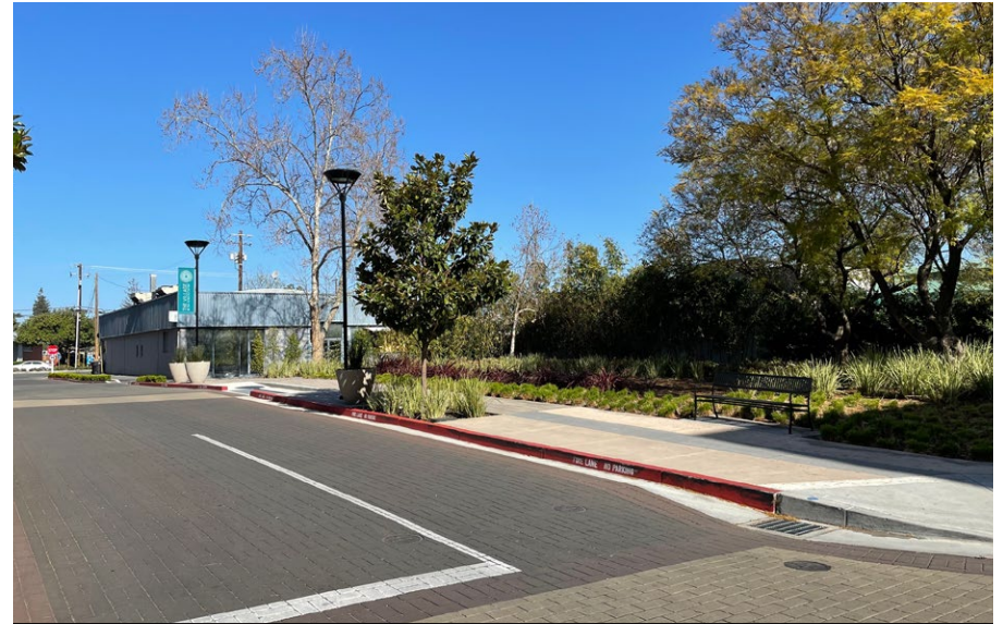
b. View of Project site from the Silicon Way and Promenade Lane intersection.
