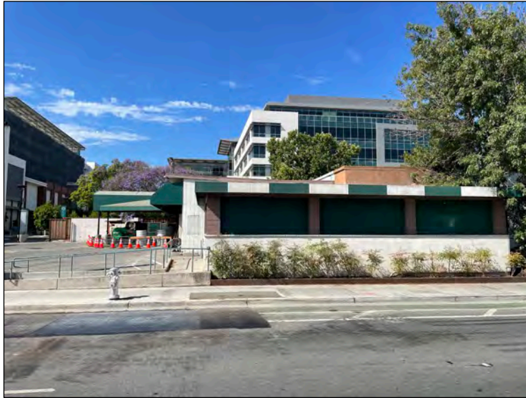
Figure 2. North façade, viewed facing south. Source: ICF.
