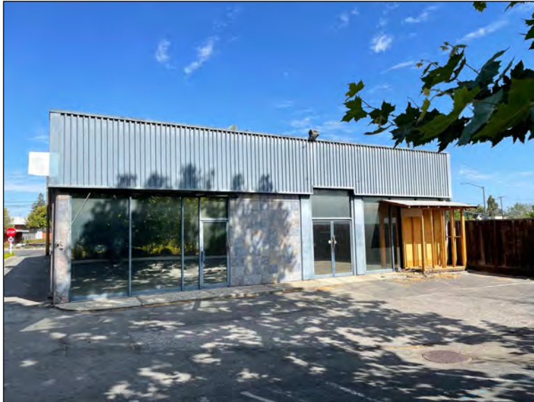
Figure 4. Rear (east) façade, viewed facing west. Source: ICF.
