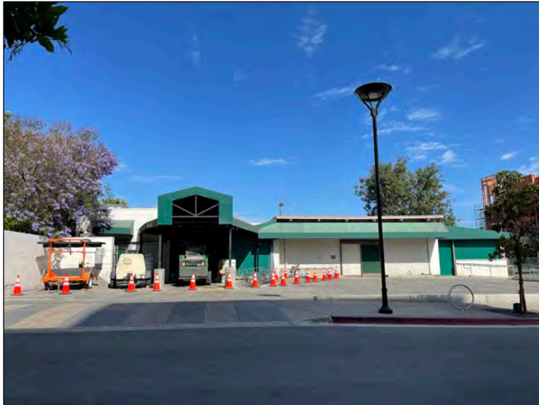
Figure 1: East façade of 2585 California Street, viewed facing west. Source: ICF.
