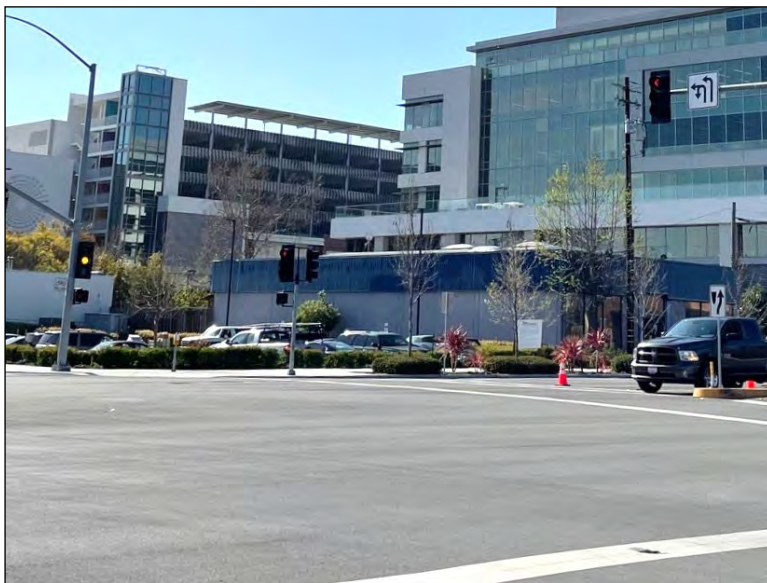
Figure 5. North façade, viewed facing southeast. Source: ICF.
