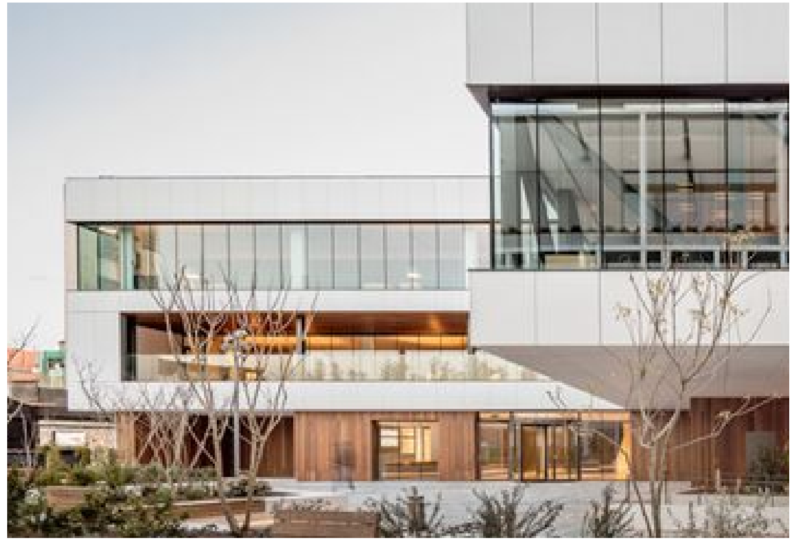
Minimal recess, clean and tight glass skin
