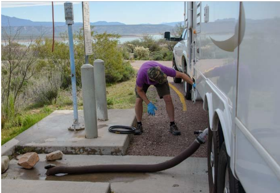
Figure 2 – Dump Station with At-Grade Sewer Connection
