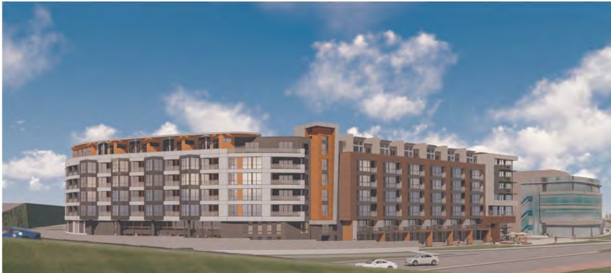
1 VIEW LOOKING NORTH WEST ON SHORELINE BLVD OVERPASS
