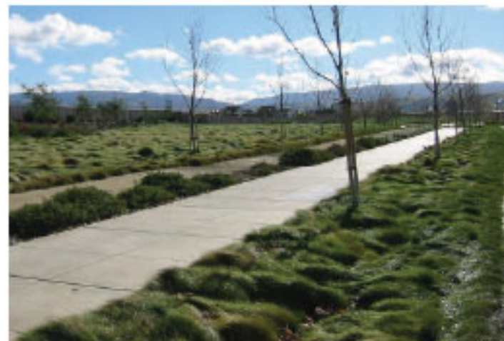
Stormwater Treatment Area
