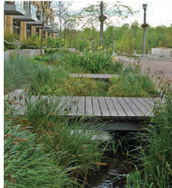
Stormwater Treatment underneath
