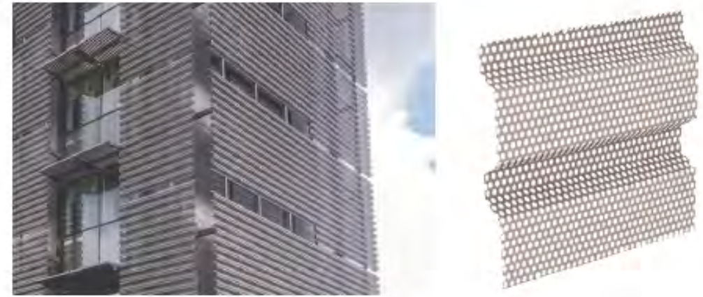
2 CORRUGATED PERFORATED METAL PANEL N.T.S.
