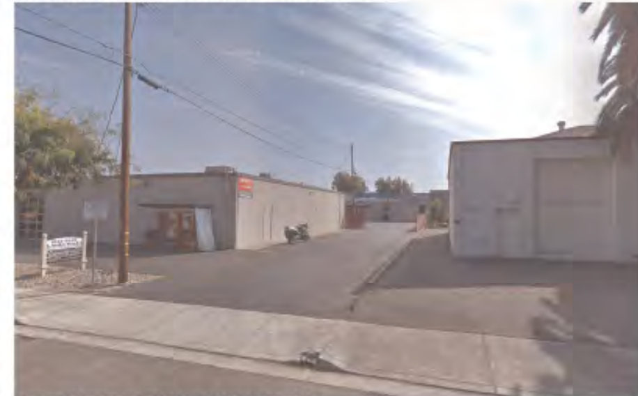
5. TERRA BELLA AVE LOOKING EAST
