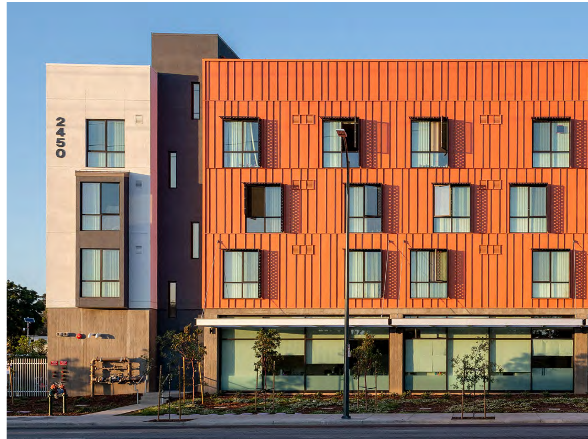
① Example of Staggered Red Oxide Board and Batten Vertical Siding
