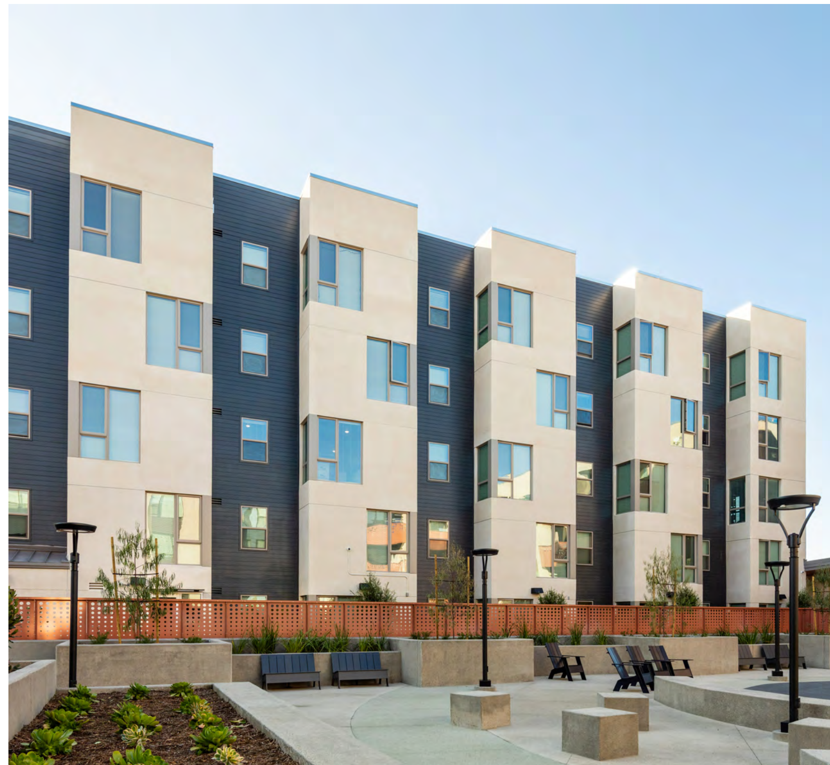
③ Plaster Wall with Jagged Parapets and Gray Accent Color (Similar to South Elevation)
