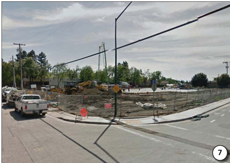
VIEW SOUTH EAST ON INIGO AND PEAR INTERSECTION
