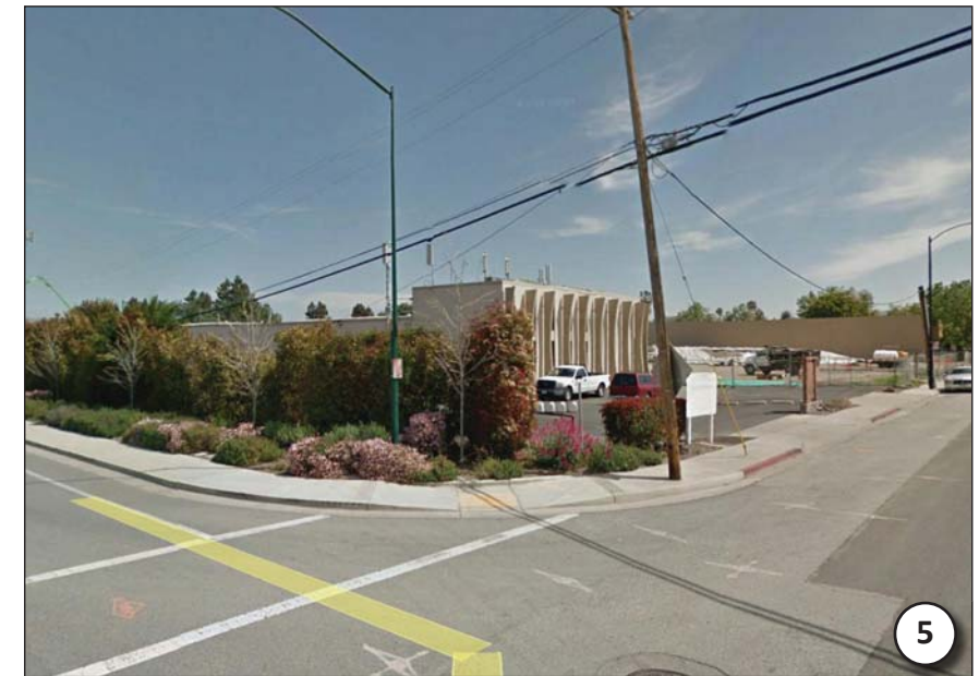
VIEW NORTH EAST ON LA AVENIDA ST
