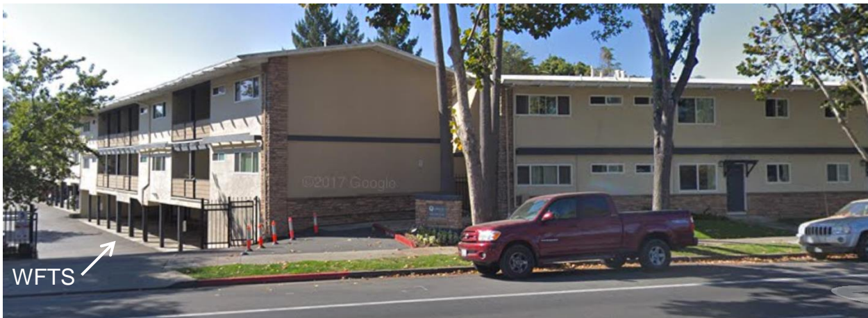
Different buildings on same parcel. Left: 3-story, WFTS, parking below grade. Right: 2-story, No WFTS
