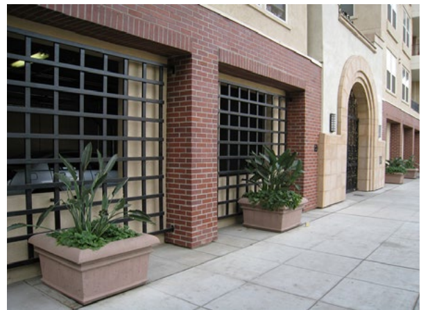
A structured podium garage with screening
