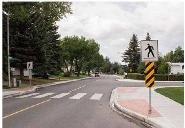
Bulb-out at crosswalk to reduce traffic speeds, improve visibility and shorten crossing distances
