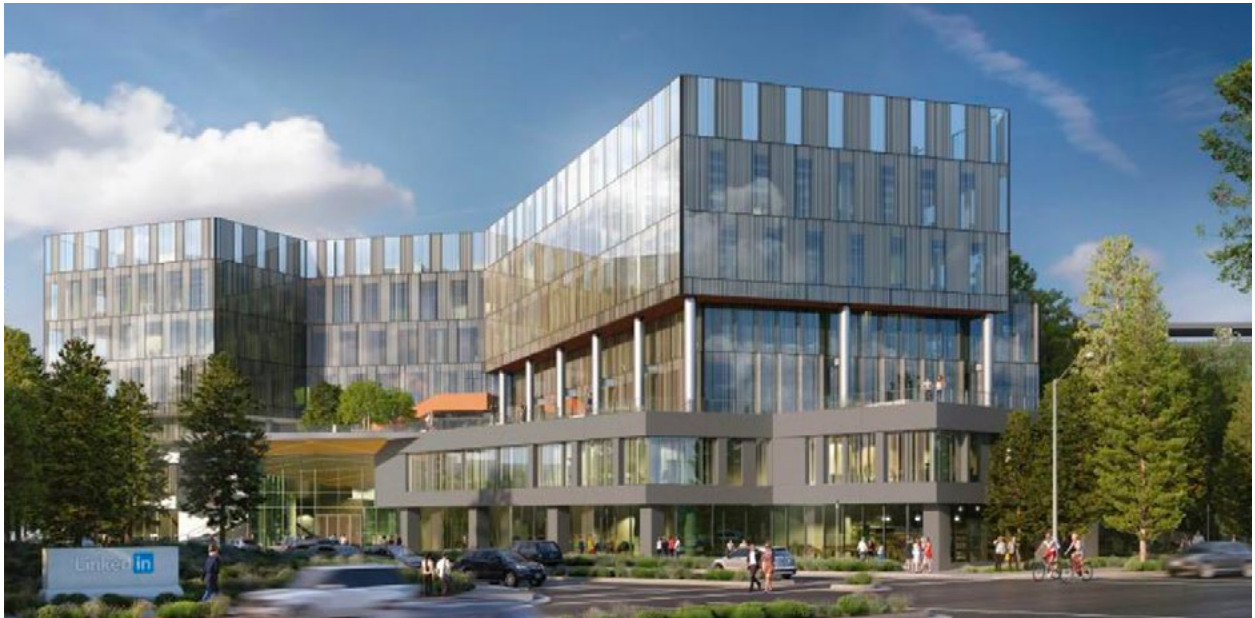
Glass curtain wall with visual interest
