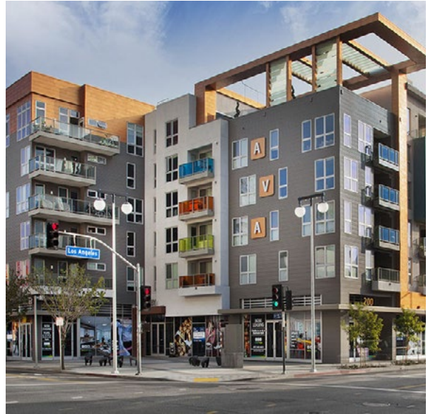
Design upper stories to reduce their bulk and mass compared to lower stories
