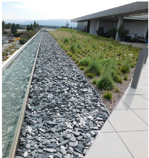
Sustainable features, such as green roofs, reduce environmental impact and create interesting building forms
