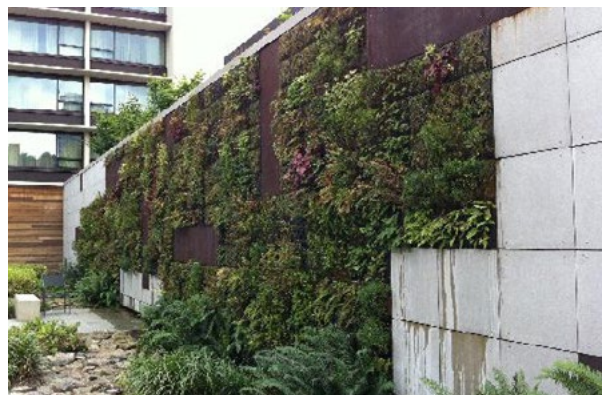
Use of landscaped green wall to screen services
