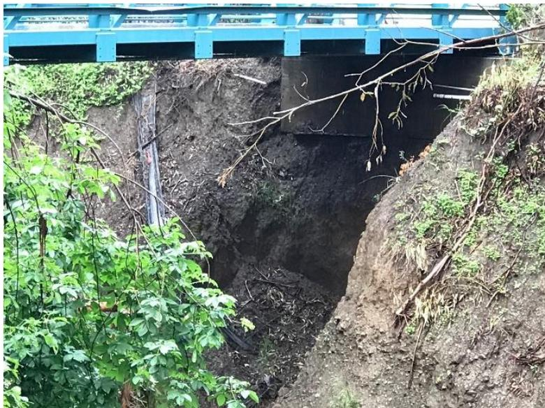
**Figure 2: Sleeper Avenue Bridge Bank Erosion**
