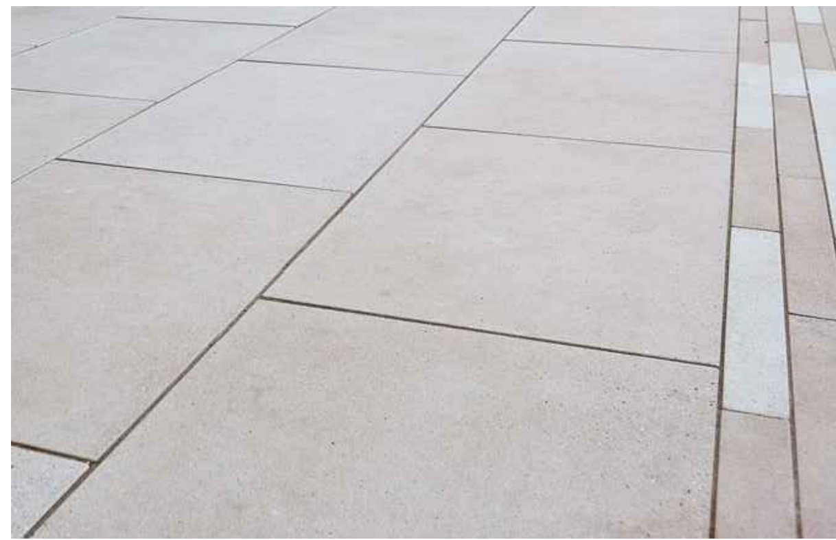
CONCRETE WITH SCORELINES TO CREATE PATTERNS
