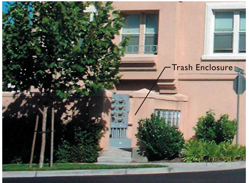
Enclosures should be located to minimize any conflict with individual units, common open space areas, or neighboring properties.
