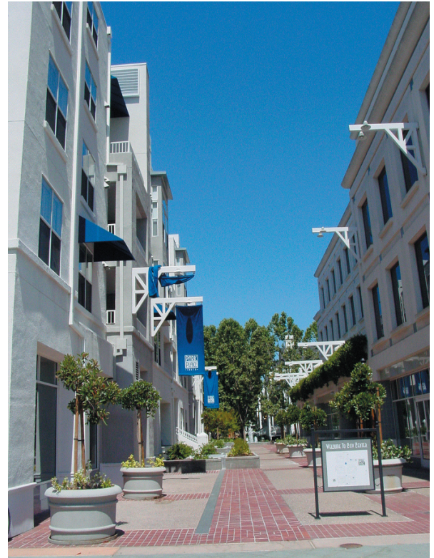
Multifamily development in the R4 zoning district shall have a maximum density of 60 80 du/ac.
