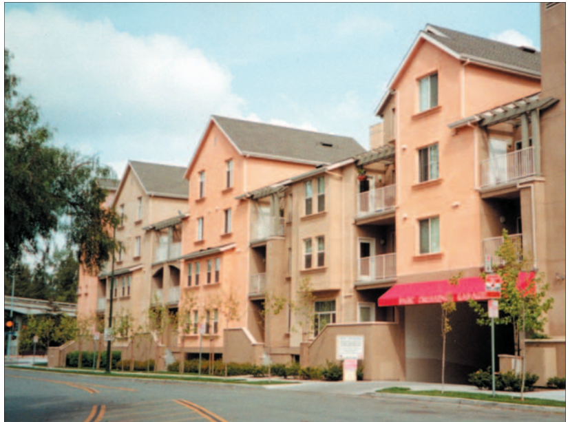
The Crossings Condominiums, an example of a high density residential project in Mountain View.
