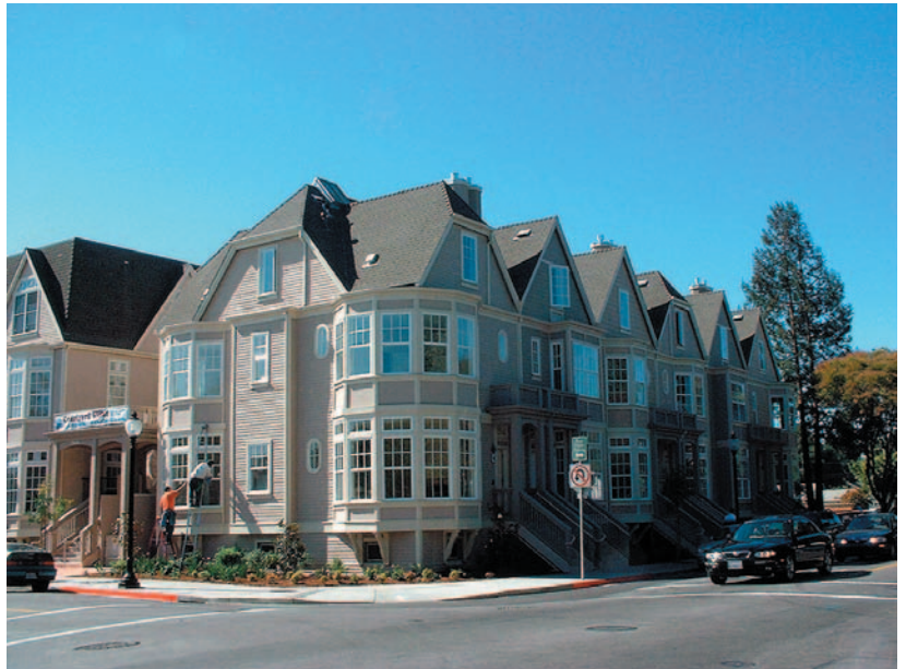
Podium Rowhouses in Downtown Mountain View
