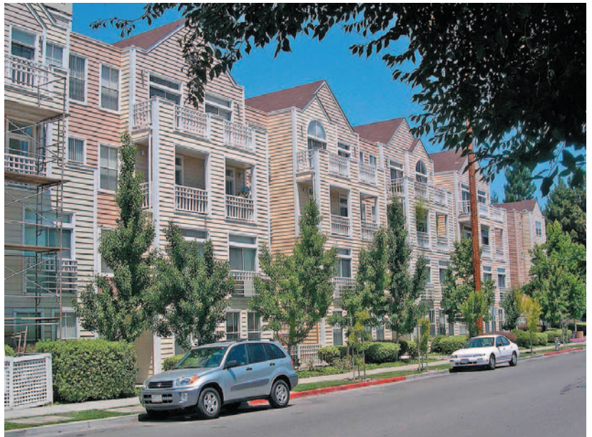
Stacked Flats in Downtown Mountain View
