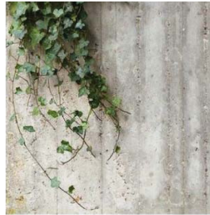
Board Formed Concrete
