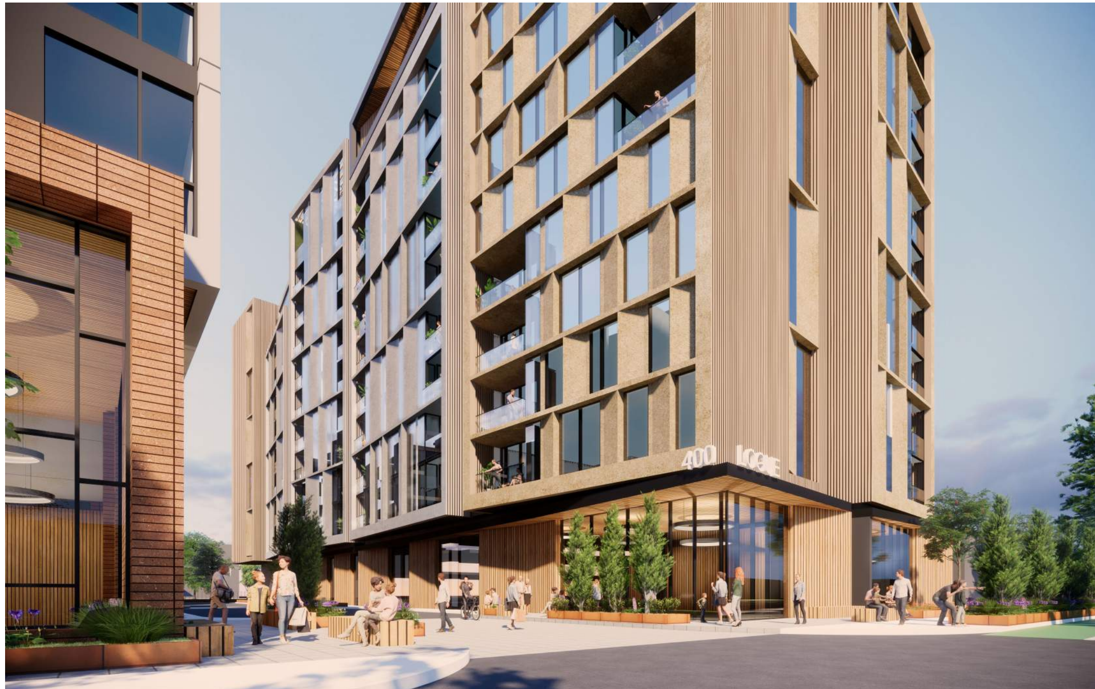
View to the Arrival Plaza, facing North. The site entrance between the two buildings is an arrival plaza landscaped with special pavers and site furnishings. Canopies, signage and glazing mark a key place in the street fabric. The arrival plaza between the two buildings provides openness and a sense of residential place mid-block.
