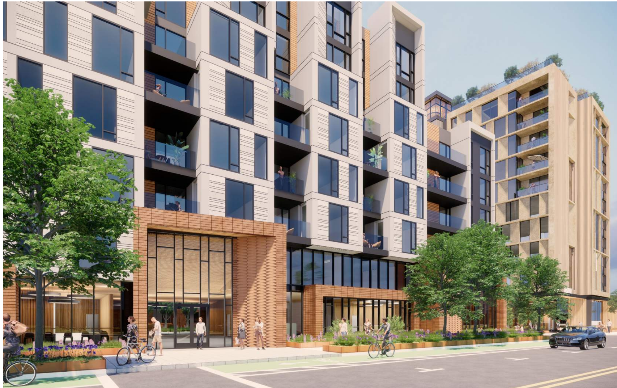
View from the Logue Avenue looking toward Building B entrance and lobby. Pedestrian circulation from Middlefield Train Station landscaped with specific tree species and integrated site furnishings such as seating and bicycle racks.
