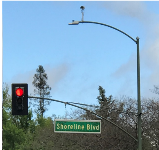
Figure 6: Existing Traffic Detection Camera that Will Need to be Updated
