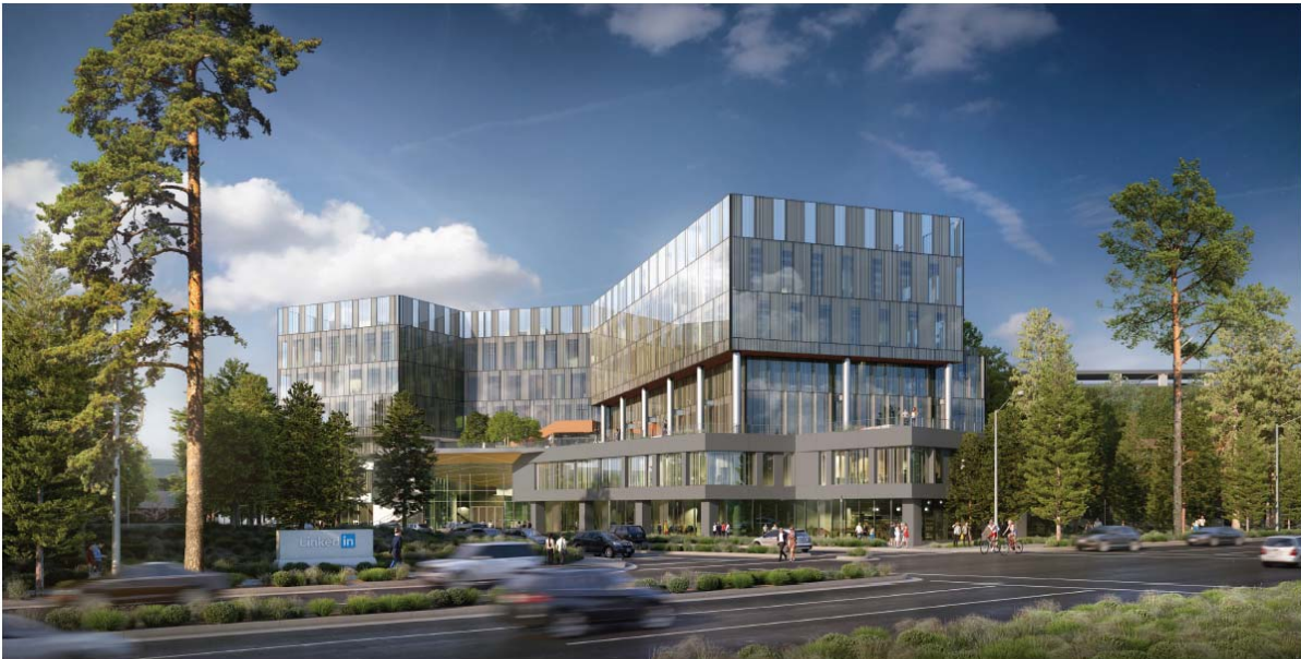
Figure 3: View of Building 1 from Bernardo Avenue
