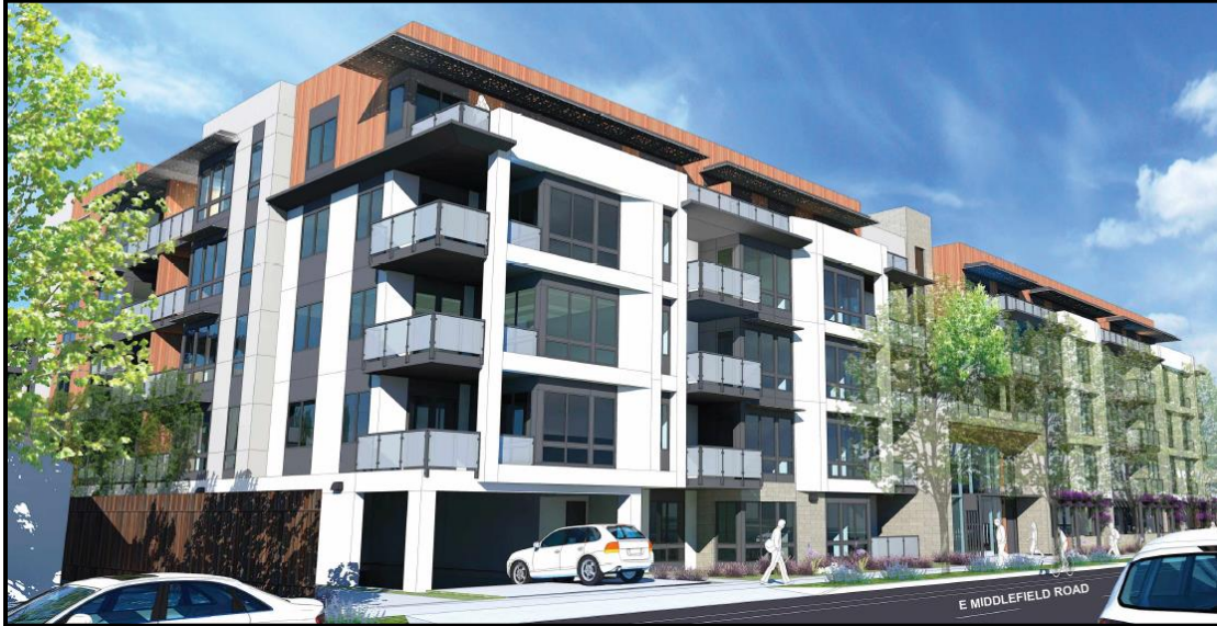
Figure 4: View from East Middlefield Road
