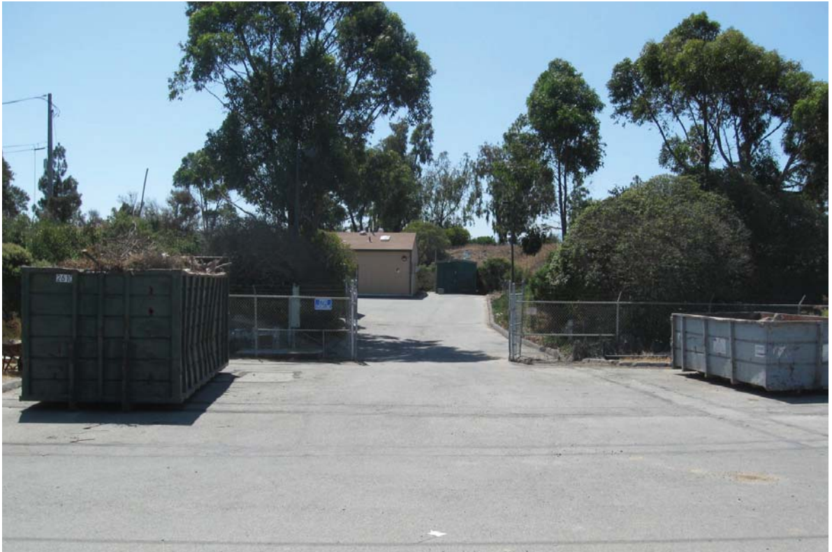
PHOTO 1: Looking south across Site B-1, showing auxiliary building and storage containers.
