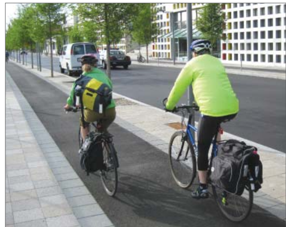
Distinctive materials can provide separation between the bicycle lane and the travel lane.
