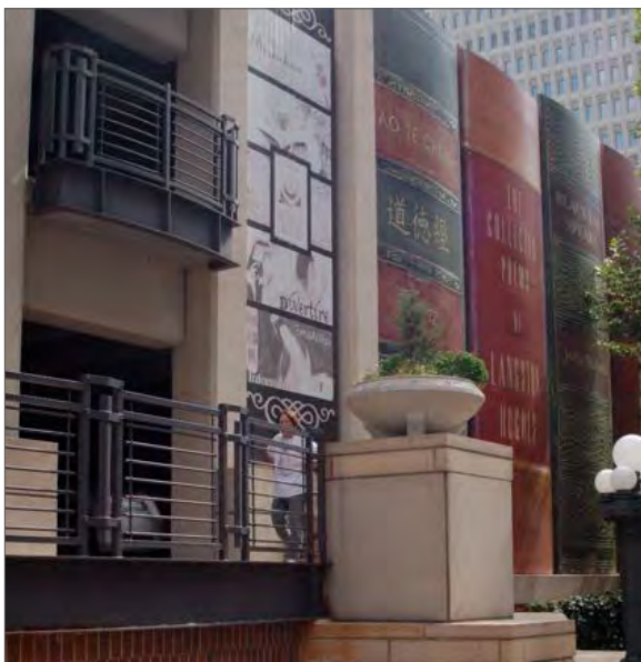
Screened parking garage.
