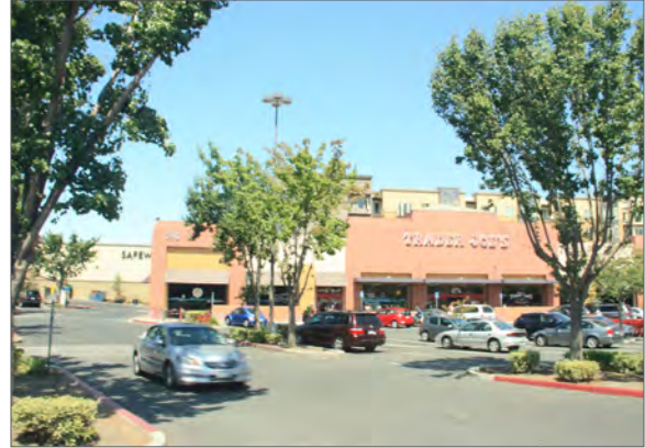
Sidewalks and pedestrian facilities are limited within the existing Center.
