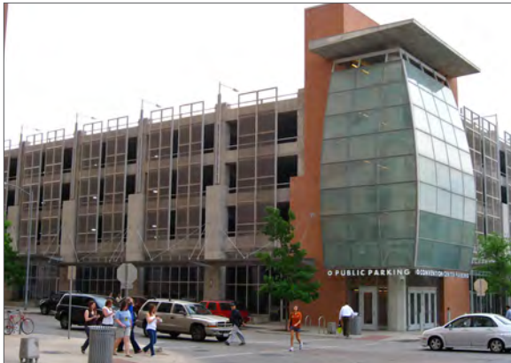
Public parking garage.
