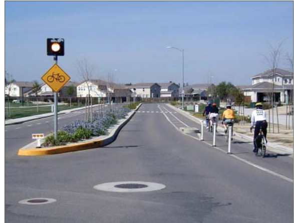
Striping of lanes, raised dividers, and painted buffers can help make bicycle lanes more visible.
