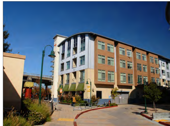
Loading area located away from main pedestrian walkway.
