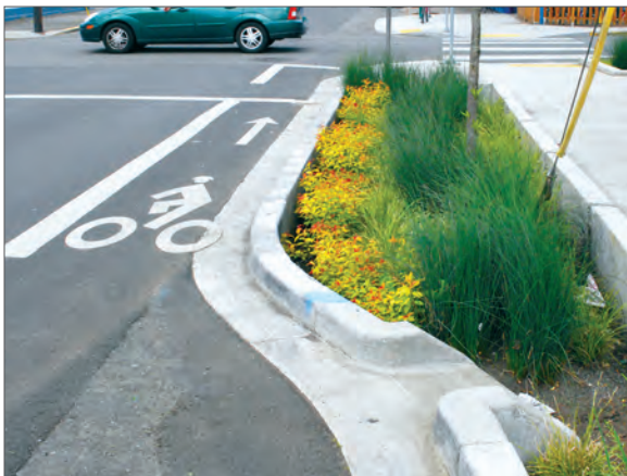
Stormwater run-off treatment.
