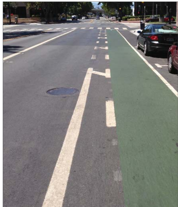
Class II bike facility with painted green lane and white buffer stripes.
