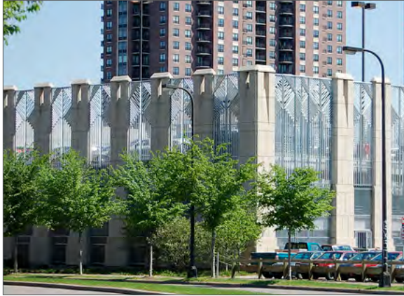
Screened parking garage.
