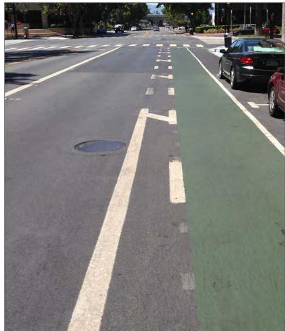
Class II bike facility with painted green lane and white buffer stripes.
