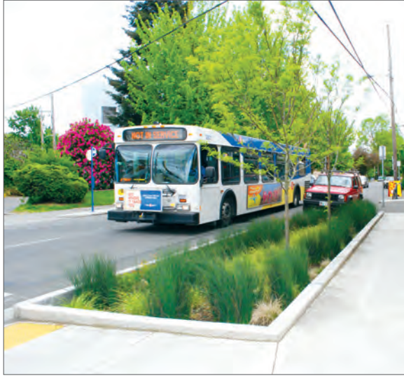
Landscaped planter zone between walk zone and bus/travel lanes, and ADA ramps at crossings.
