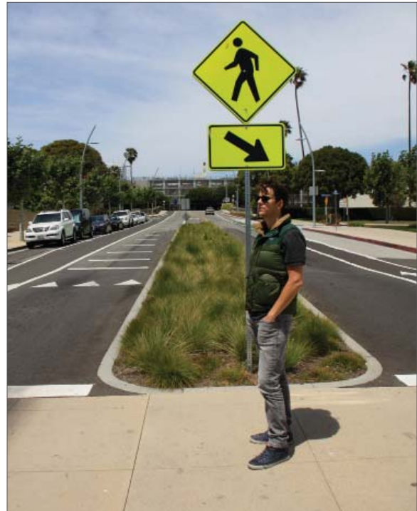
Mid-block pedestrian crossing with landscaped median, pedestrian refuge, and signage to alert drivers.
