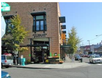
Least Favored Ground-Floor Character and Least Favored Overall Building Shape (tie)
