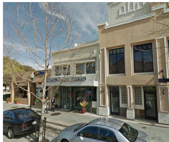
Example of Small Project Sites
