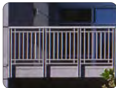
METAL BALCONY RAILING
