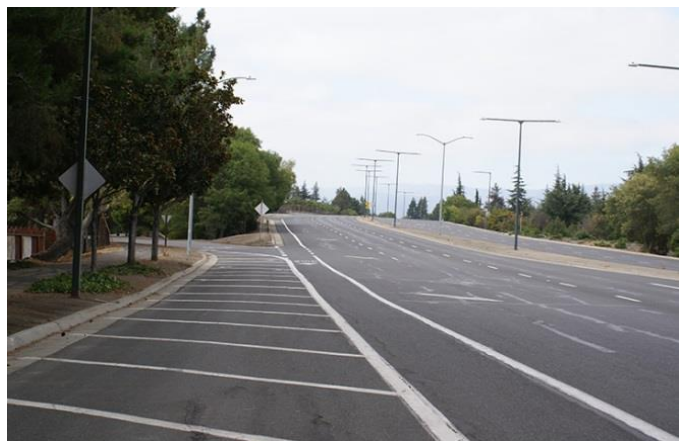
Figure 2— Shoreline Boulevard at Central Expressway
