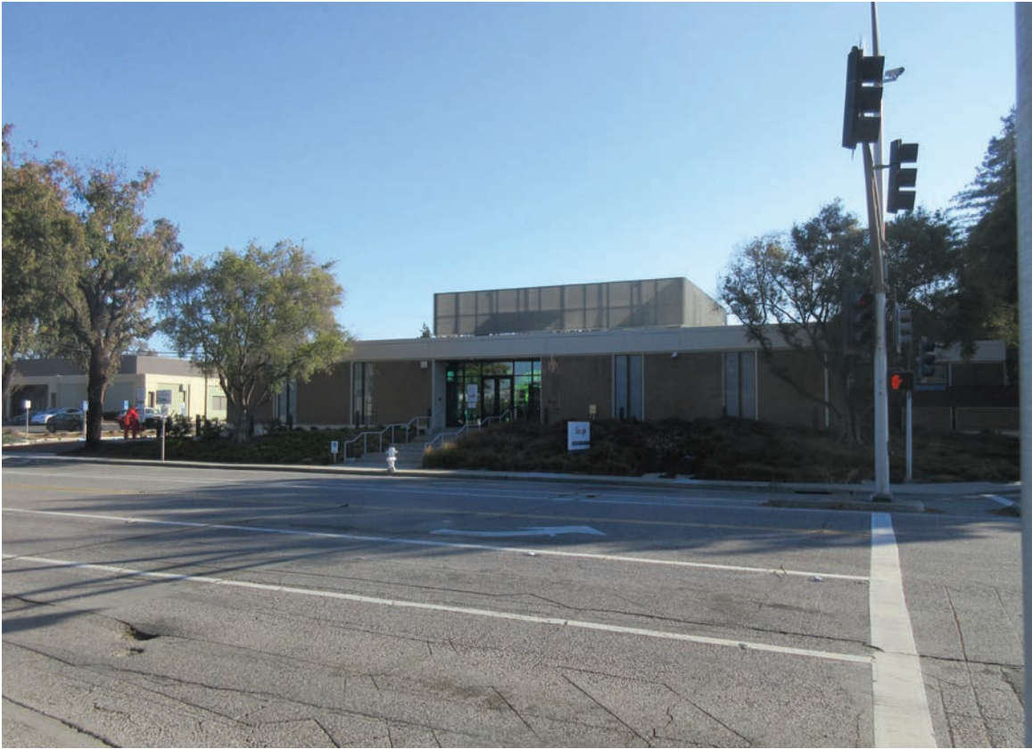
Photo 1: View from the northeast corner of the San Antonio Road and Bayshore Parkway intersection looking east towards the project site.
