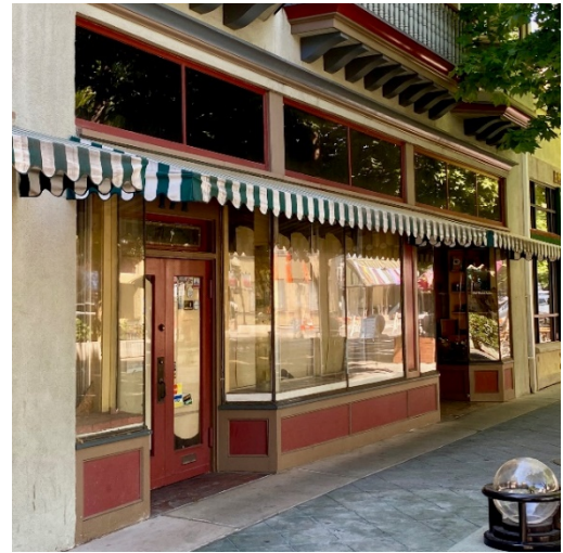
Fig. H.9: Entry alcove at street-facing building facade
