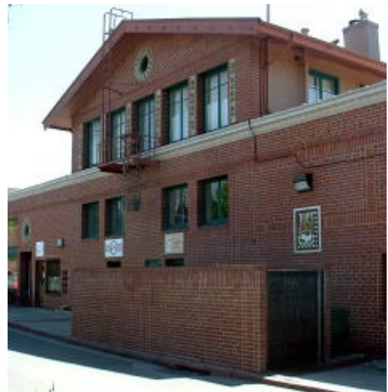
Fig. H.19: Service facilities should be screened with enclosures and devices consistent with the building architecture.
