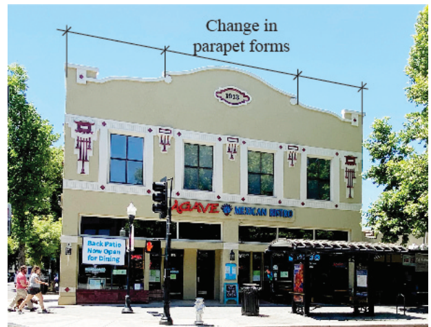
Fig. A.10: Interesting roof forms are encouraged throughout the downtown.
