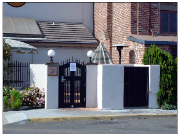
Fig. H.26: Trash and loading areas should be well screened from view in structures that are consistent with the building design in both materials and detailing.
