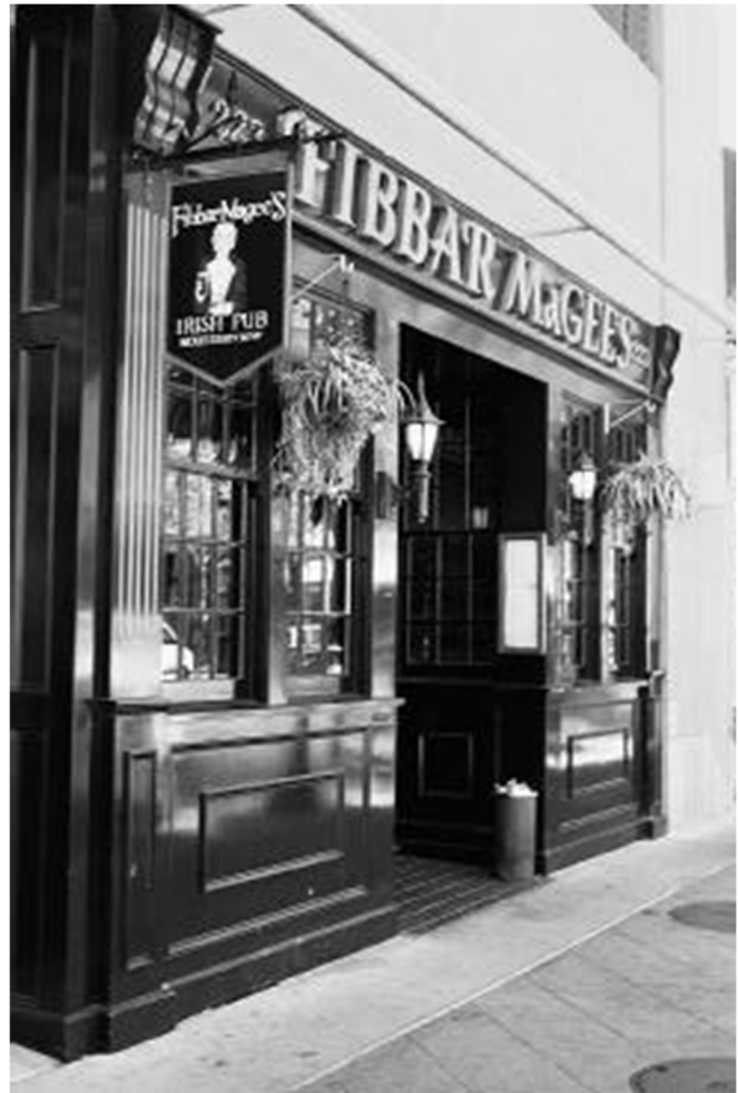
Fig. H.23: New storefront renovation on Castro Street. Entrances should be recessed from the facade, creating a small alcove.
