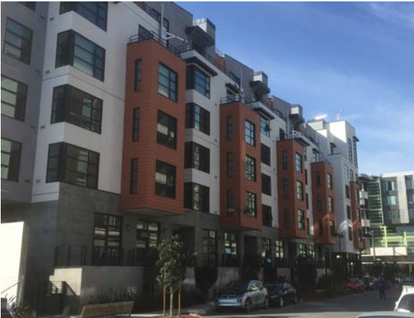
Vertical massing of residential buildings is accentuated with smaller scale vertical elements, emphasizing their height and access to light and views
