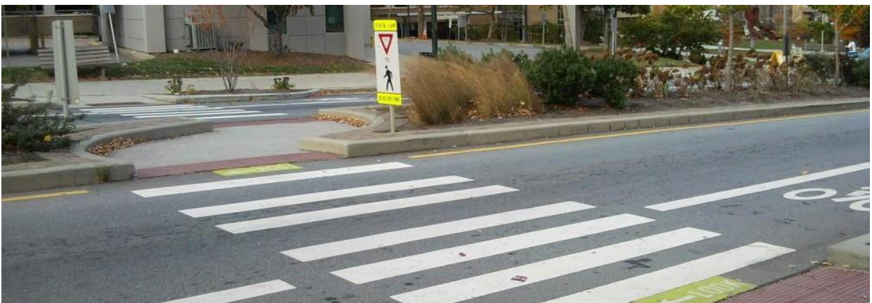
Example of mid-block crosswalk
