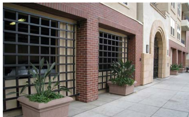
A structured podium garage with screening
