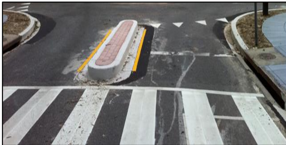
Figure 8 – Example of Splitter Island
