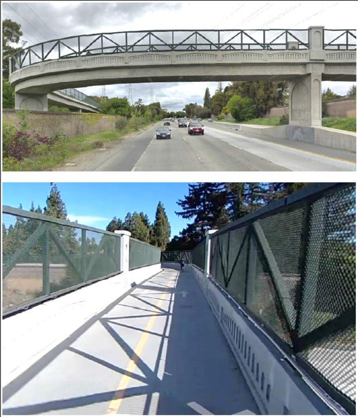
Figure 13: Mountain View Stevens Creek Trail Bridge
