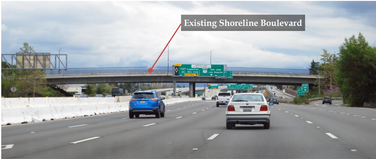
Figure 9: Street View Southbound Highway 101 Approaching Shoreline Boulevard
