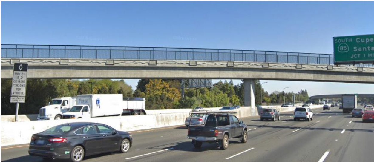
Figure 12: Mountain View Permanente Creek Trail Bridge
