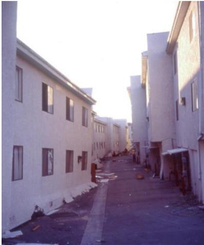
1C. Left: Collapsed 3-story building. Right: Sidesway damage, Los Angeles, Northridge earthquake (Credit: Gary D. Avey)
