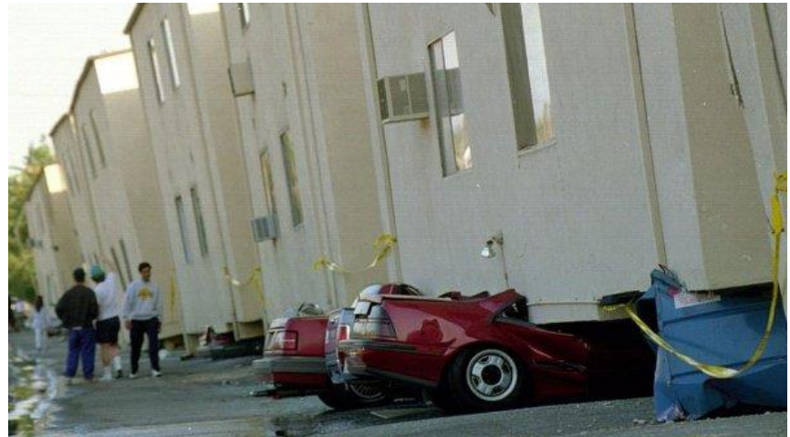
Collapsed 3-story building, Los Angeles, Northridge earthquake (Credit: Boris Yaro, Los Angeles Times)
