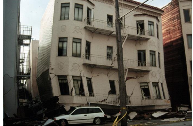
Collapsed 4-story building, San Francisco, Loma Prieta earthquake
