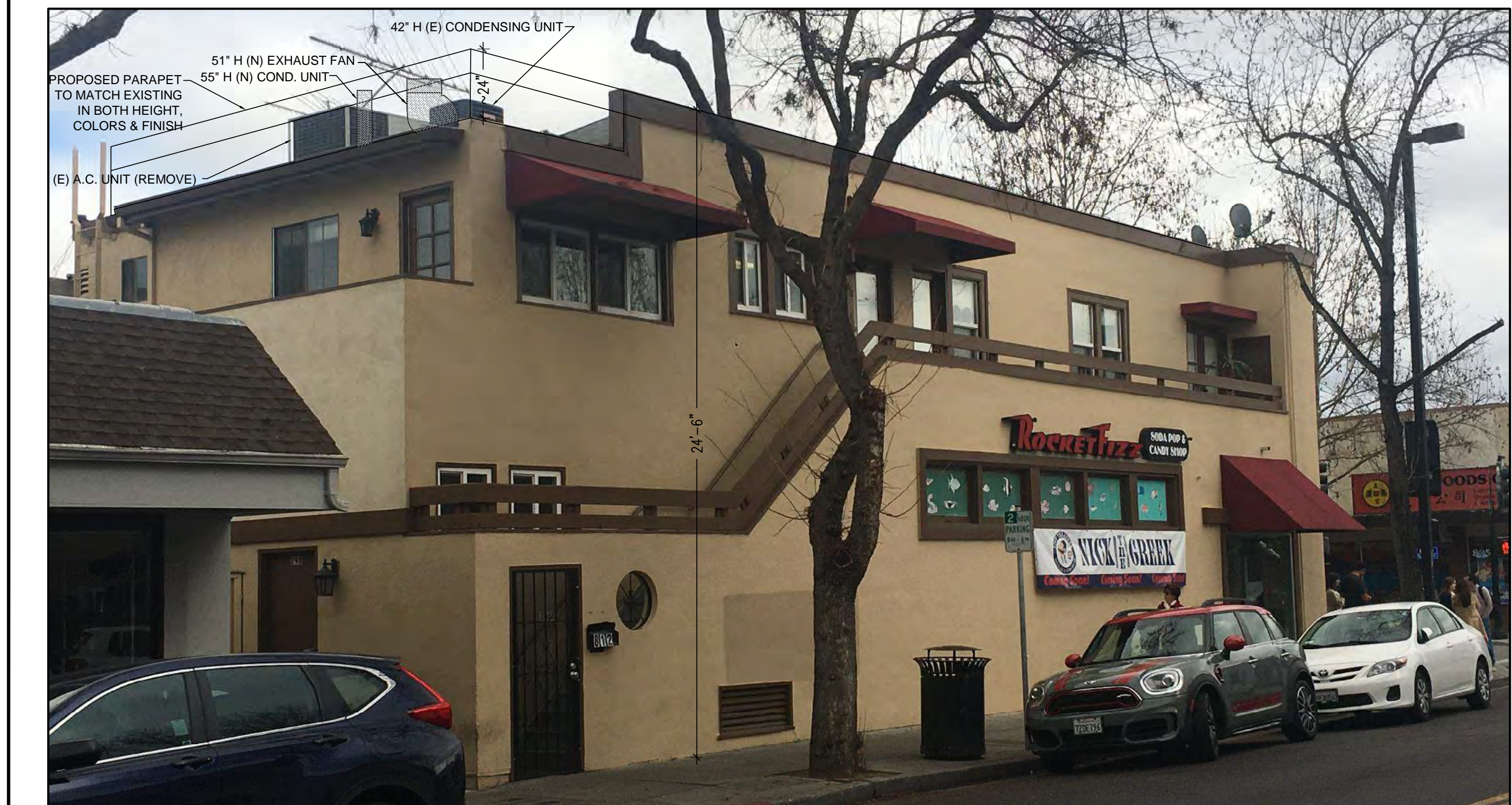
4 VIEW FROM SOUTH-WEST (FROM SIDEWALK WEST ACROSS W. DANA STREET)
