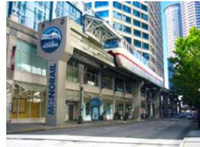
Seattle Monorail Guideway
