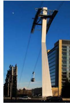
Portland Aerial Tram and Cable Guideway Tower
