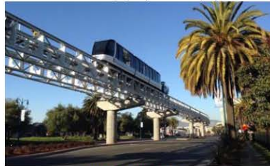
Oakland Airport Connector APM Guideway
