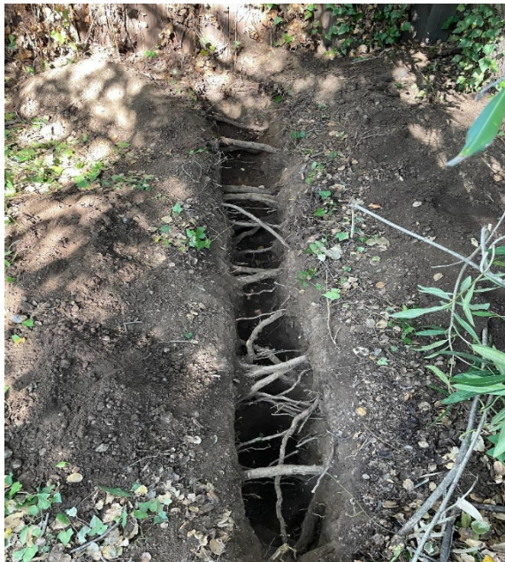
Showing trench at 6.5' from trees
