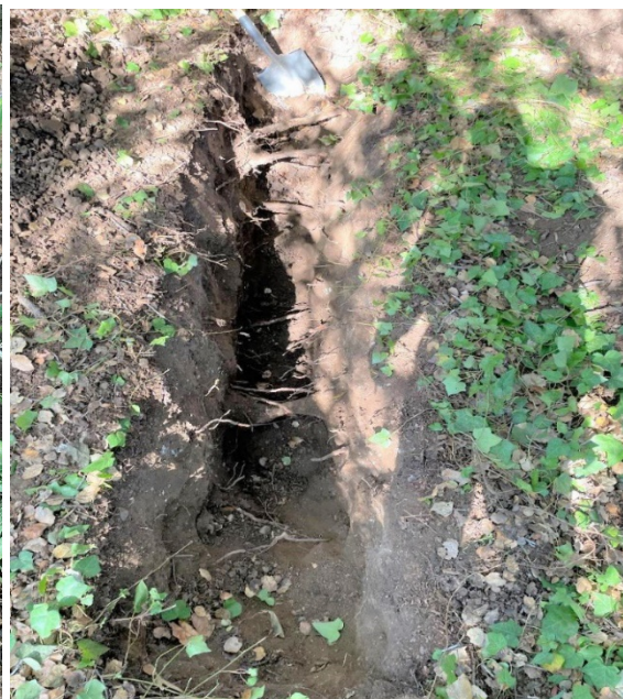
Showing trench at 9.4' from trees
