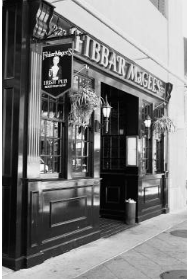
New storefront renovation on Castro Street. Entrances should be recessed from the facade, creating a small alcove.
