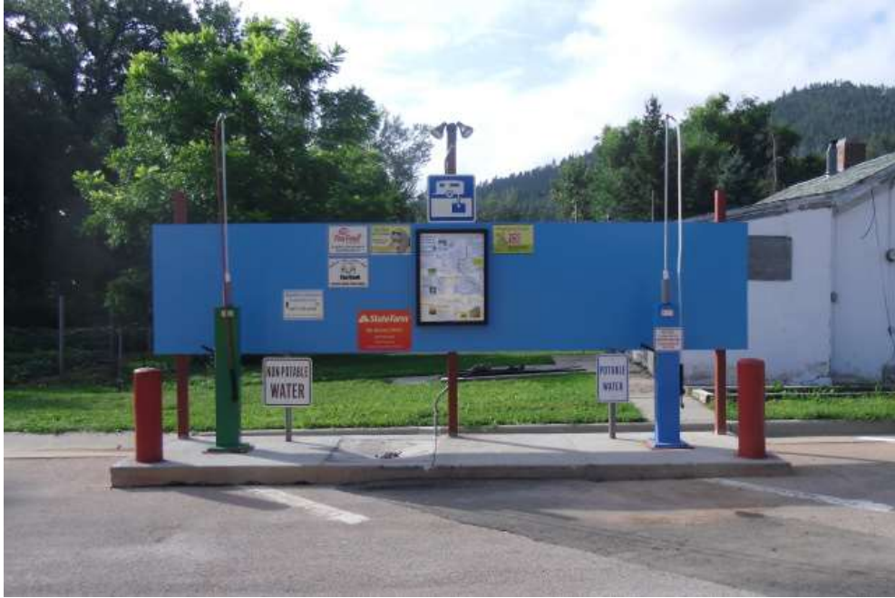
Figure 1 – Dump Station with Waste Disposal and Water Towers in Raised Concrete Pad
