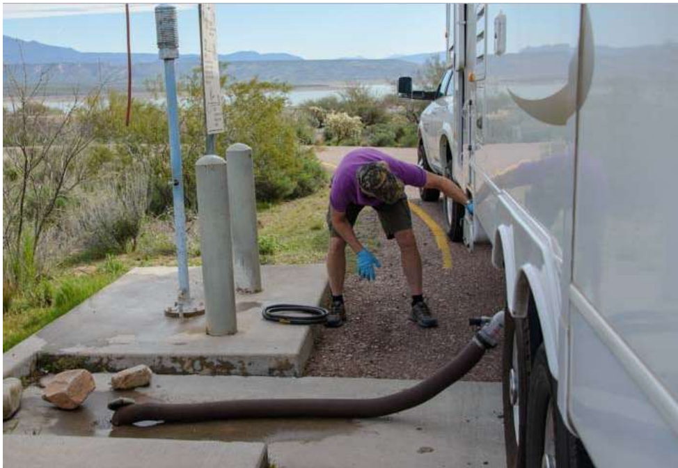
Figure 2 – Dump Station with At-Grade Sewer Connection
