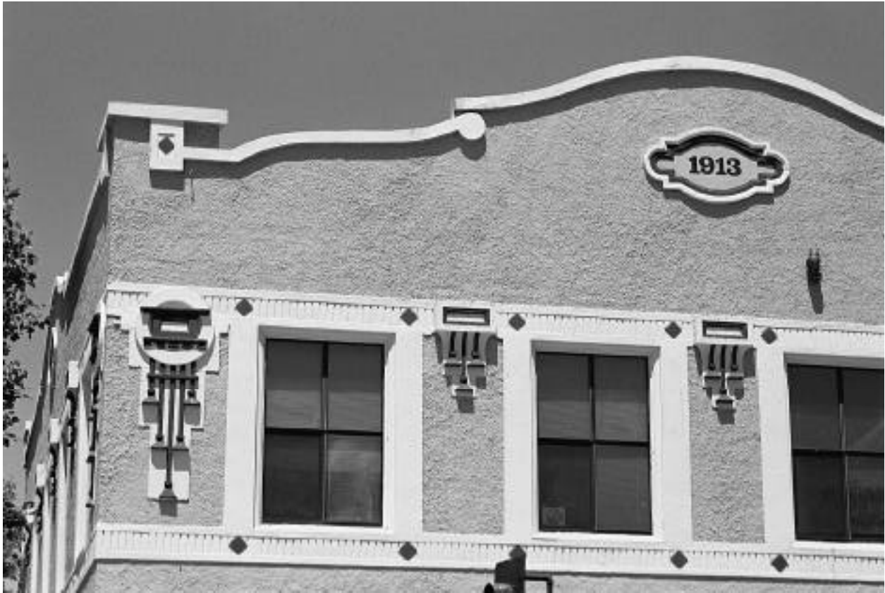
The Jurian Building, originally constructed in 1913.
