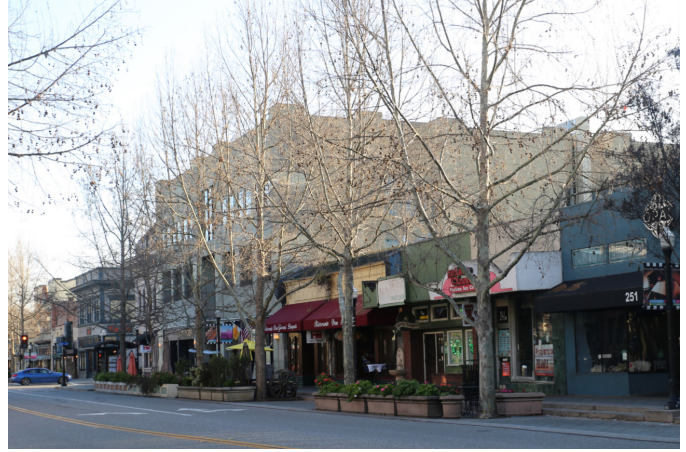
Storefronts along Castro Street — human scaled with layers of landscape.
