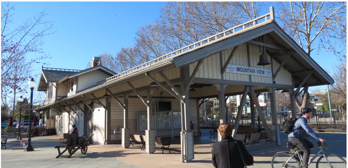
Downtown Mountain View Station is served by Santa Clara VTA light rail and Caltrain regional rail service.
