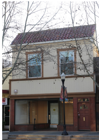
Intimate scale of existing buildings.
