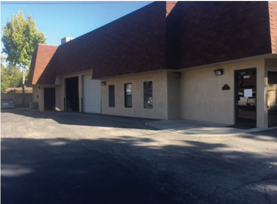
Photo 2: View of the warehouse building on-site on Colony Street.
