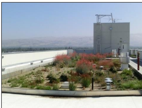
Figure 2-7: Green roof at Fourth Street Apartments, San José. (Source: EOA)
