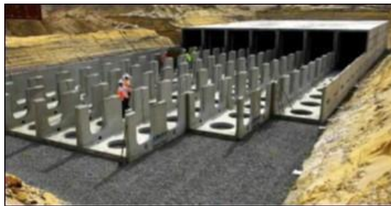
Figure 2-12: Subsurface vault, under construction. (Source: Conteches.com)
