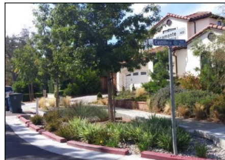
Figure 2-2: Bioretention in curb extension, Southgate Neighborhood, Palo Alto (Source: EOA, Inc.)
