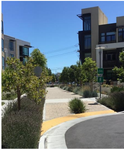
Figure 5-1: Pervious paving installed at a public walkway connecting Stierlin Road and the Central Expressway/Castro Street intersection, which was constructed as part of a regulated project. (Source: City of Mountain View)
