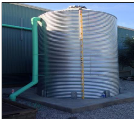
Figure 2-8 Rainwater harvesting cistern, Environmental Innovation Center, San José (Source: City of San Jose)
