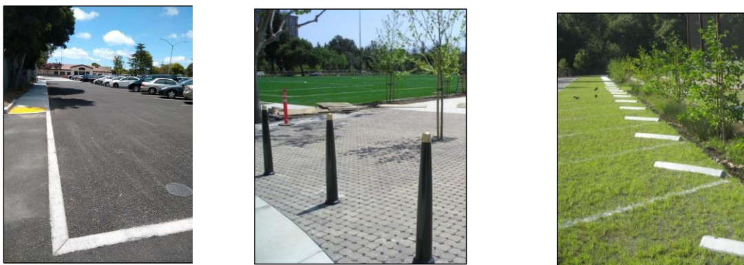
Figure 2-4: Permeable asphalt, Turner Court, Alameda (left, source: EOA, Inc.); permeable interlocking concrete pavers, Mayfield Playing Fields, Palo Alto (middle, source: EOA, Inc.); parking stalls constructed with recycled plastic geocells filled with special soil and planted with turf grass, Cupertino (right, Source: City of Cupertino).
