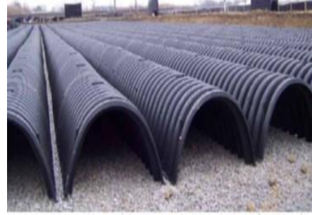
Figure 2-6: Subsurface infiltration system, under construction (Source: Conteches.com )
