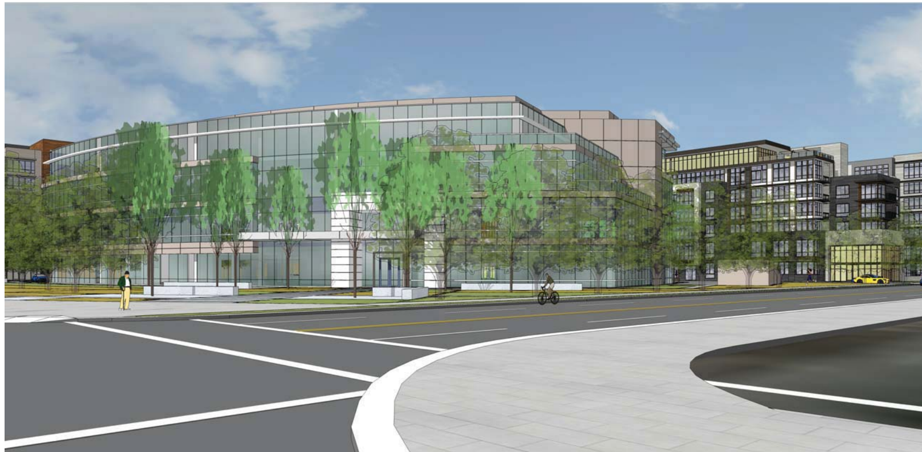
VIEW 4 : Perspective View on N Shoreline BLVD at Terra Bella Ave Looking from West to East
