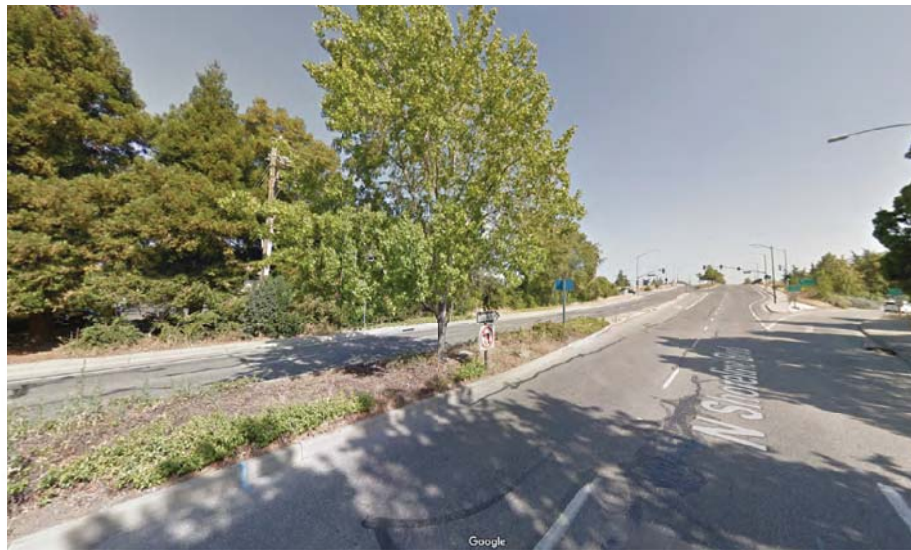
2. NORTH SHORELINE LOOKING NORTH WEST
