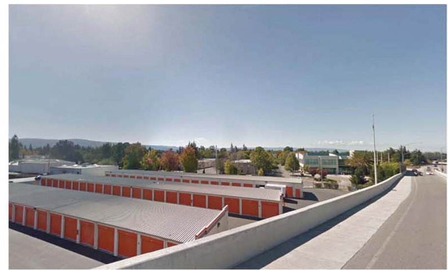
4. US 101 FREEWAY LOOKING SOUTH WEST
