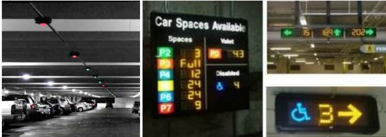
Figure 1-9: M3 Park Assist Guidance System (with per-level occupancy signs)
