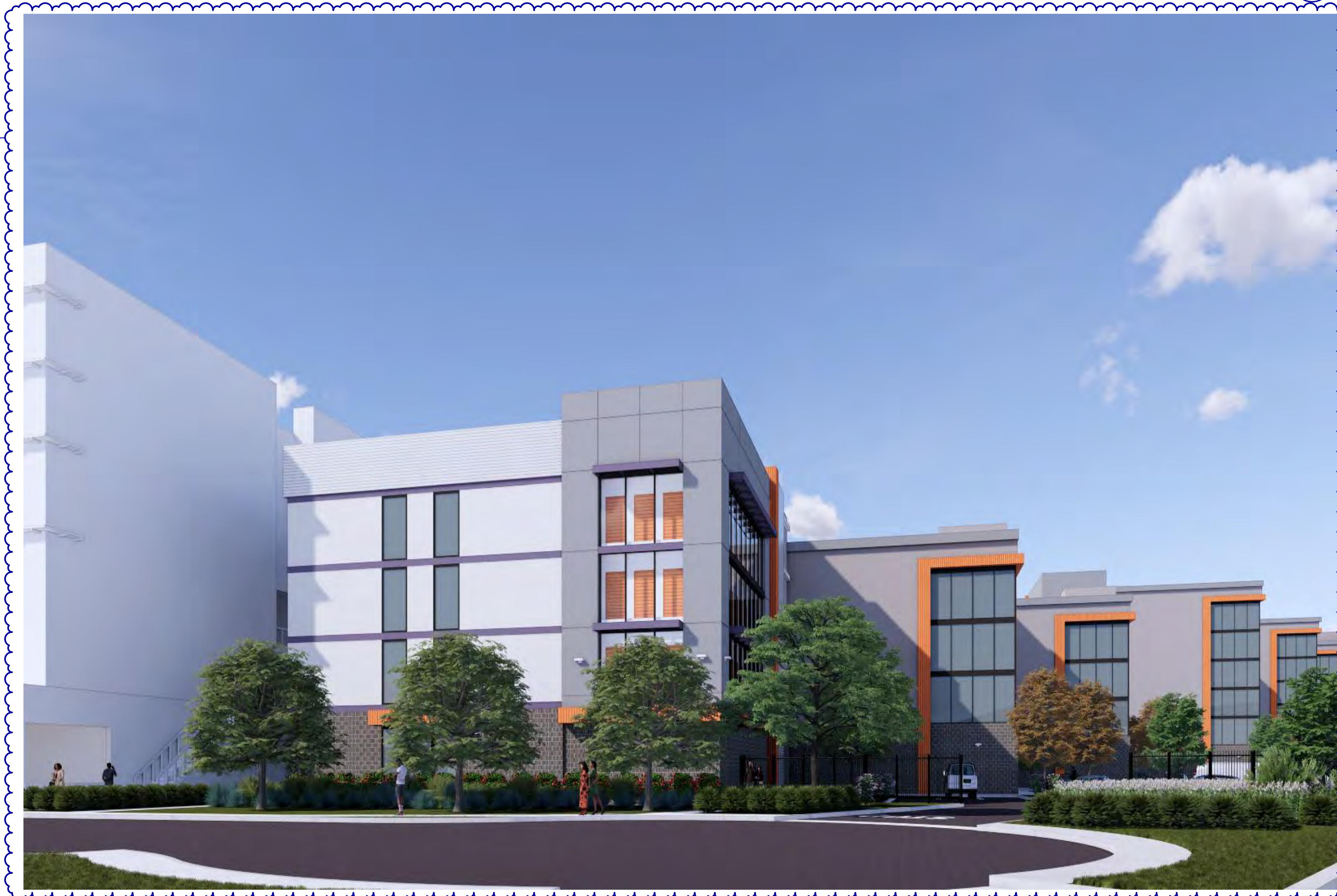
BUILDING 1 - SW CORNER VIEW
